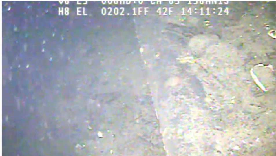
Figure 4 Sedimentation on north side of pipe, indicating strong bottom currents
