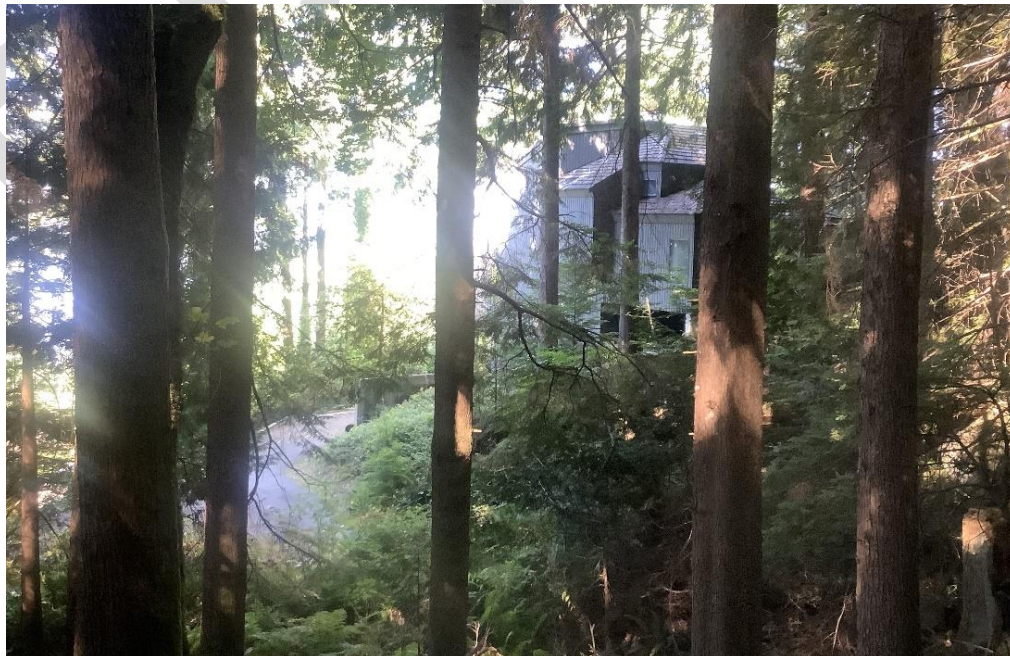
Photo 15. Example of a structure in the interface
