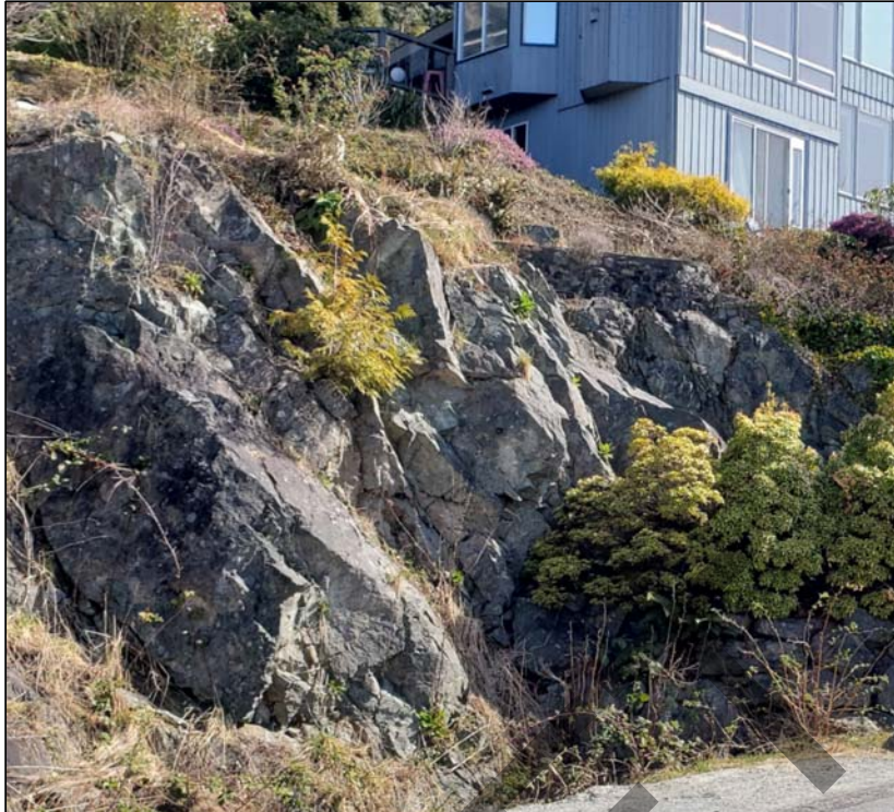
Photograph 6: closer view of exposed bedrock discontinuities.
