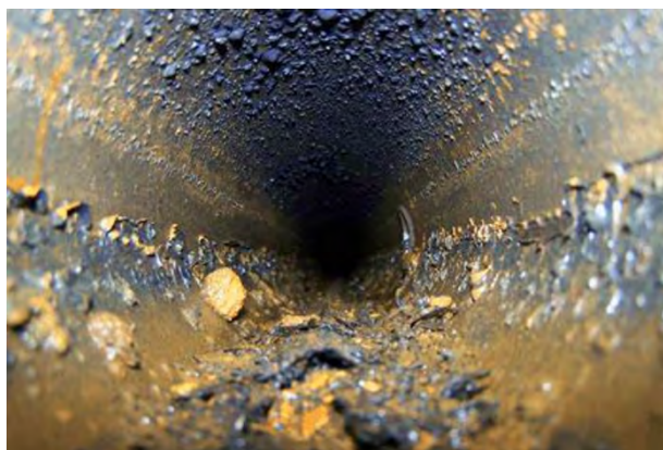
Debris buildup and biofilm formation within a section of ductile iron water main
