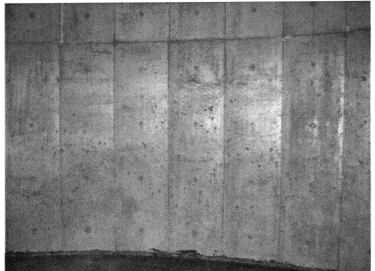
159. Tank wall viewed from the inside to be in good condition
