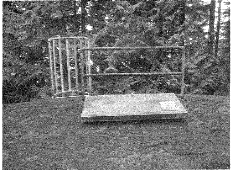
68. Access hatch and guardrail
