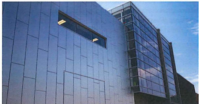
The new Mount Pleasant Substation will be the first LEED-standard substation in BC Hydro's system.
