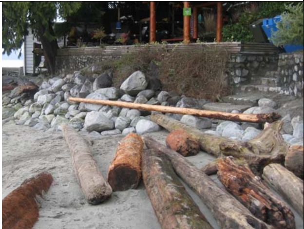
Photo illustrating example of loose rocks at base of wall as added protection.
