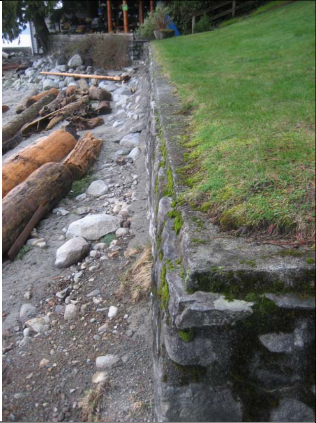
Photograph noting vertical and horizontal alignment – seems intact, i.e. no lean.
