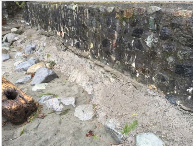
This photo shows an area that has been previously reinforced with cement and embedded rocks.
