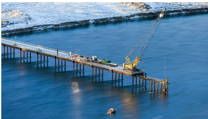
The 329-metre Peace River construction bridge was completed in March 2016, linking the north and south banks of the dam site.
