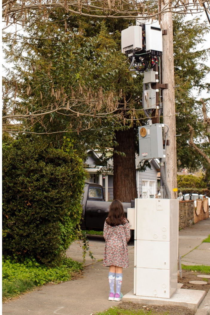
Microcell Installation in Santa Rosa, California
