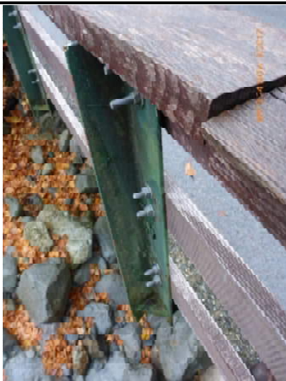
007 – Top rail misalignment; deformed post (5 th from North on East side)
