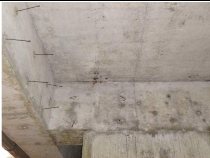
015 – Pier 1, typical delaminations at Pier to Soffit interface with rust staining.
