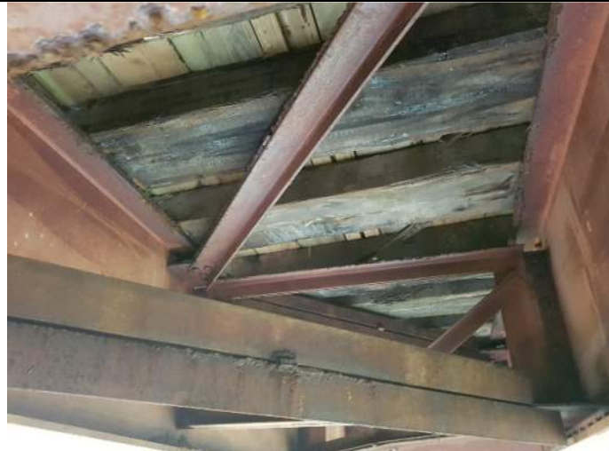
014 – Bearing at North Abutment. Note severe crushing.
