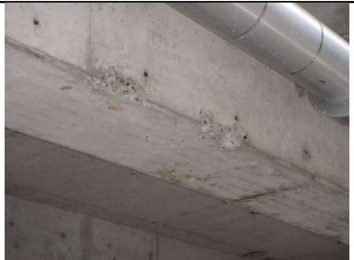
014 – Light Spalling from impact damage on Girder 1 midspan
