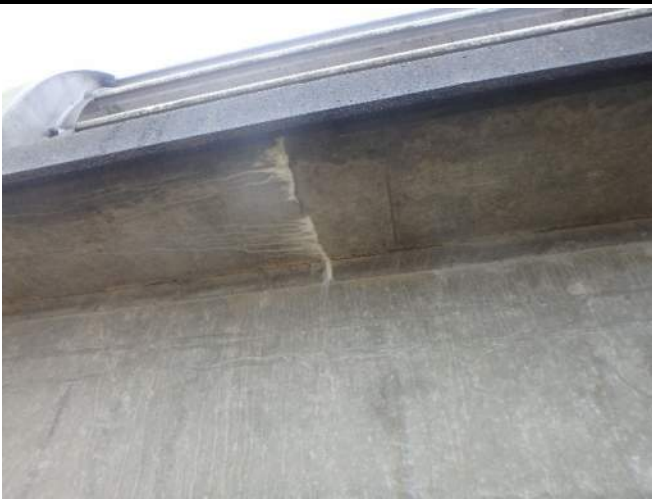
019 – Transverse cracks with efflorescence on the underside of curb typical.
