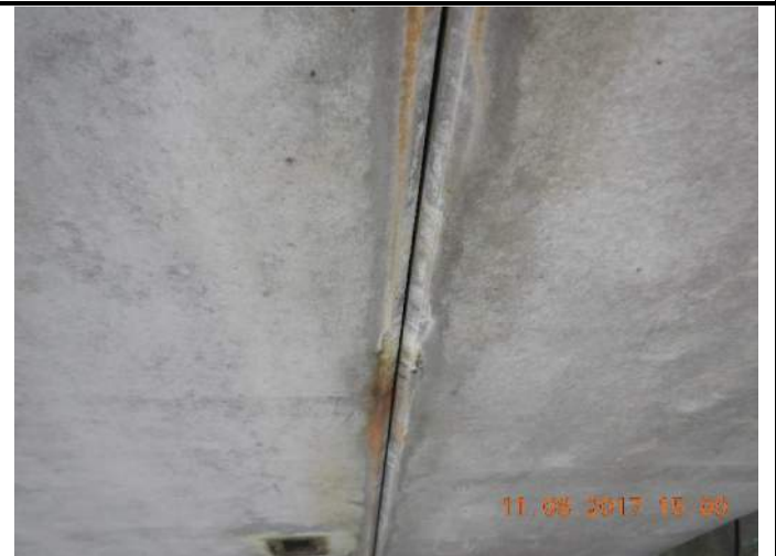
028 - Leaking between girders
