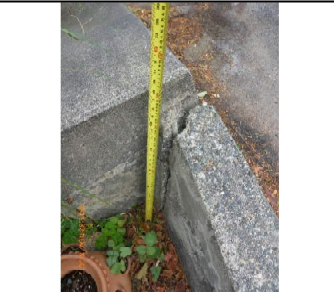
005 – Barrier detached at South-West corner
