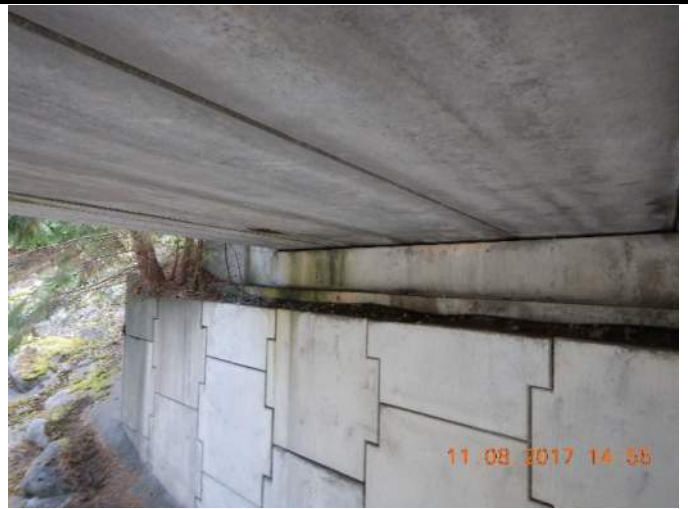
024 – South Abutment: efflorescence deposits, water leaking signs, horizontal cracks with rusting
