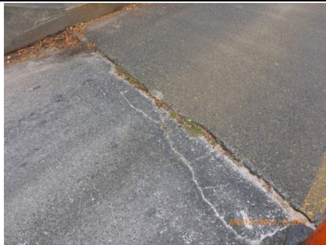
003 – Asphalt cracking at South Approach
