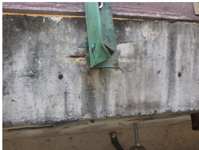
008 – Deformation at the bottom of the post (5 th from North on East side)
