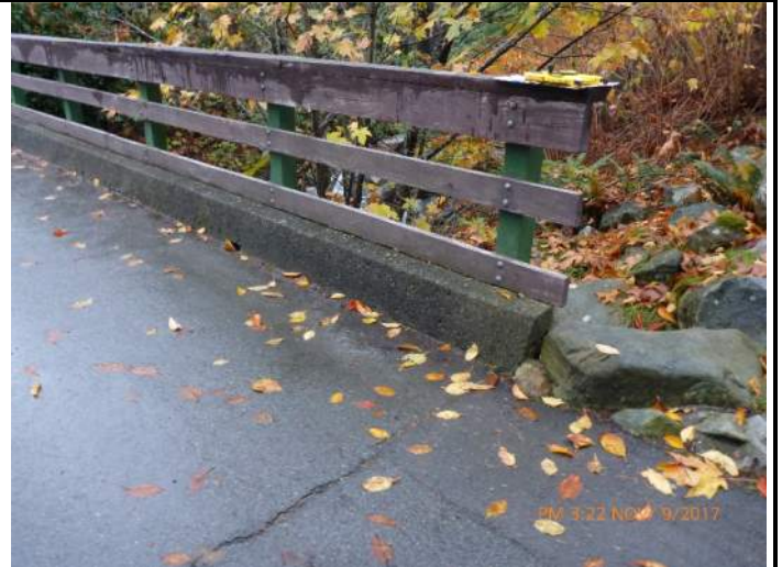
002 – Delamination area at SE corner of the deck
