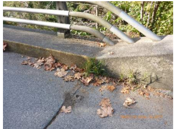
004 – Scaling on deck NW corner
