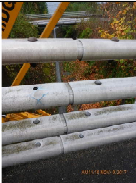
007 – Missing splice bolt at West side railing
