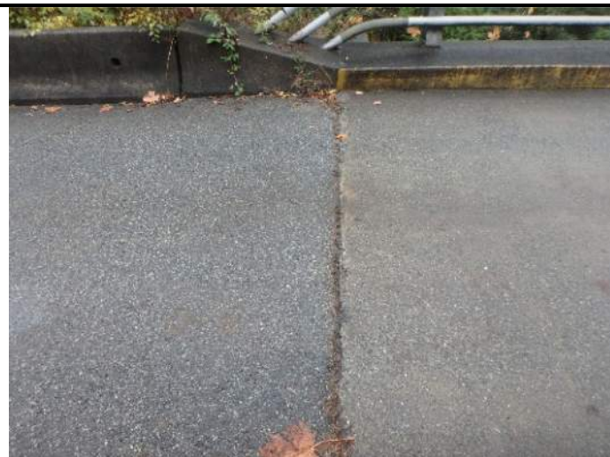
002 – Typical gap between deck and approach
