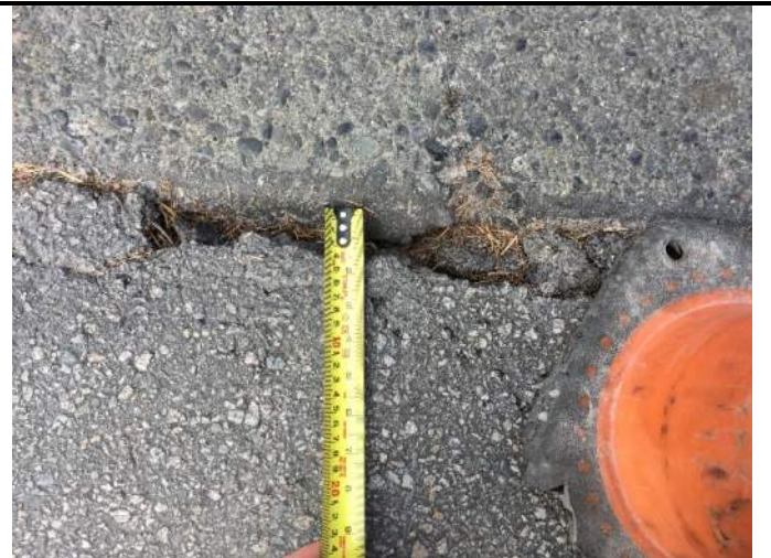
006 – Spalls in asphalt on South approach
