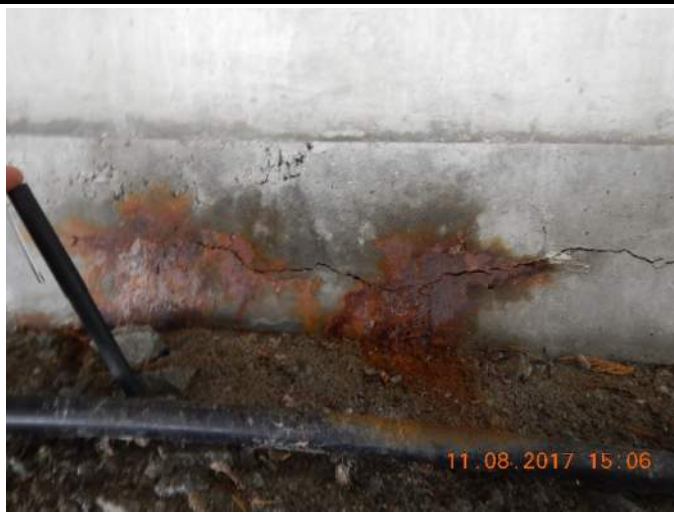
025 – South Abutment: horizontal cracks with rust staining
