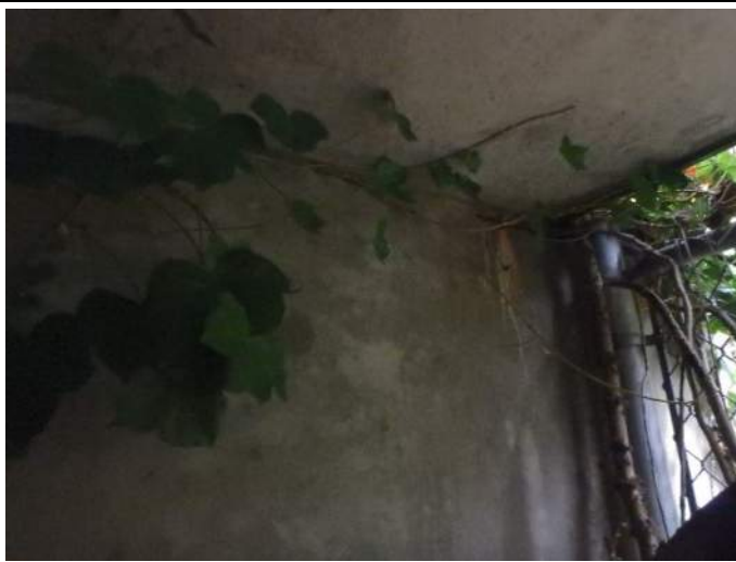
013 – Vegetation growth between abutment wall and underside of girders.
