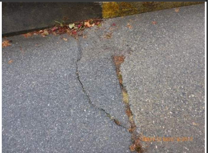
004 – Crack in asphalt at South approach, West side
