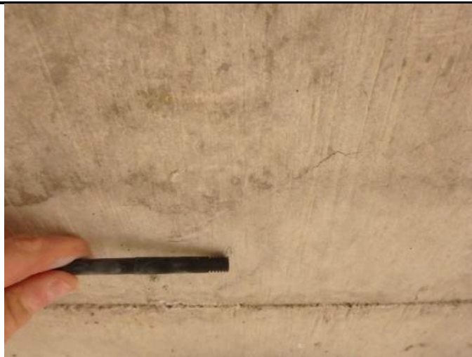
013 – Hairline cracks at soffit, typical
