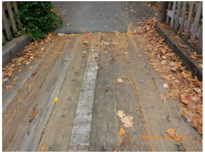
008 – Normal wearing at deck with minor checking
