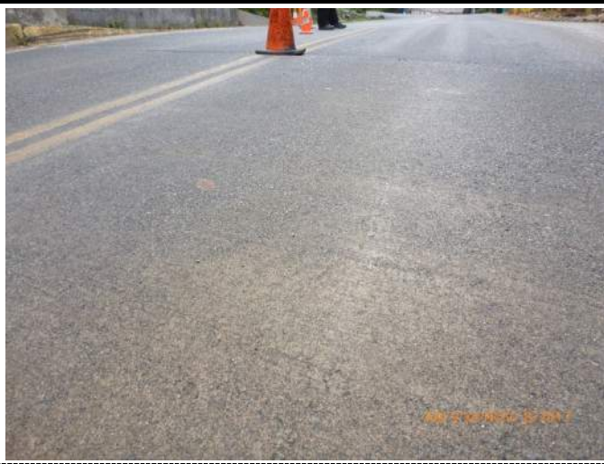
007 – Longitudinal hairline crack at SB lane (similar at NB lane)
