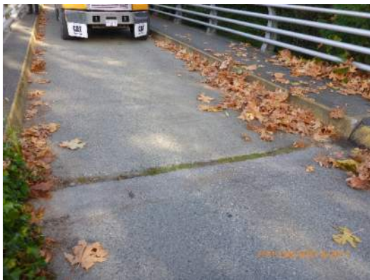
005 – South Approach gap between deck and asphalt
