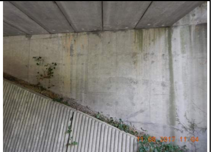
012 – South Abutment: evidence of leaking at West side, localized medium delamination under Girders 4 and 5
