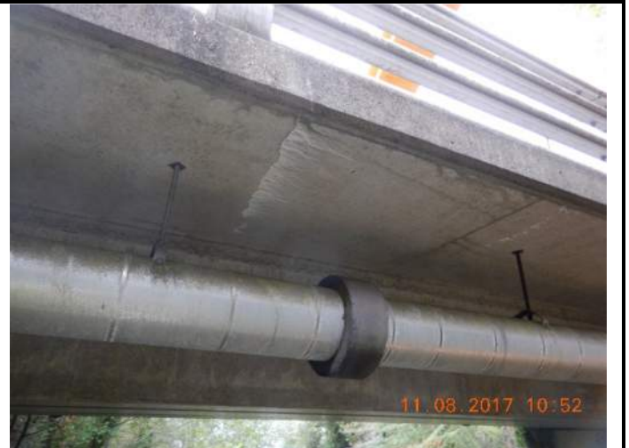
018 – Typical transverse cracks with efflorescence on the underside of sidewalk
