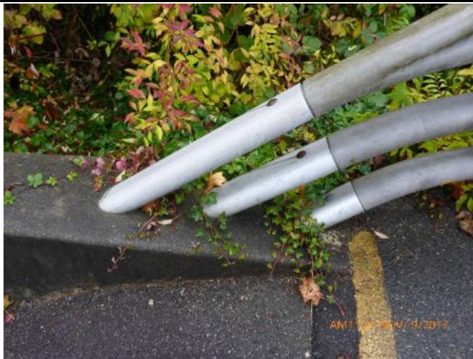
009 – Rusty bolts at the railing, typical
