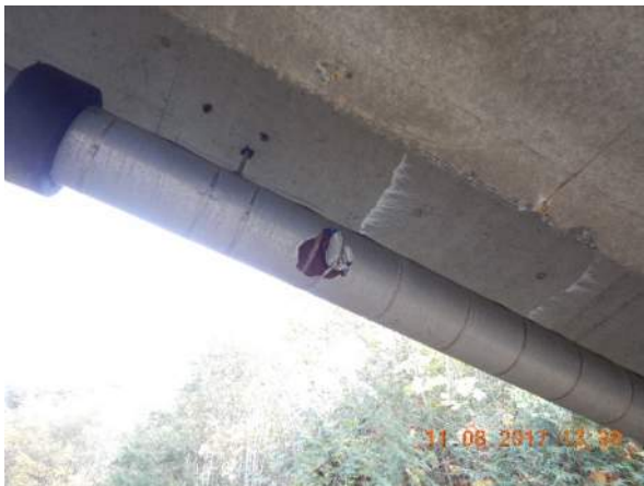
017 – Damage at watermain cover
