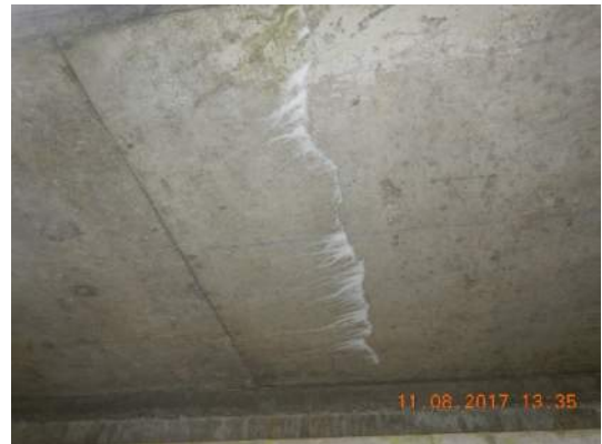
018 – Transverse cracks with efflorescence on underside of sidewalk and curb typical.
