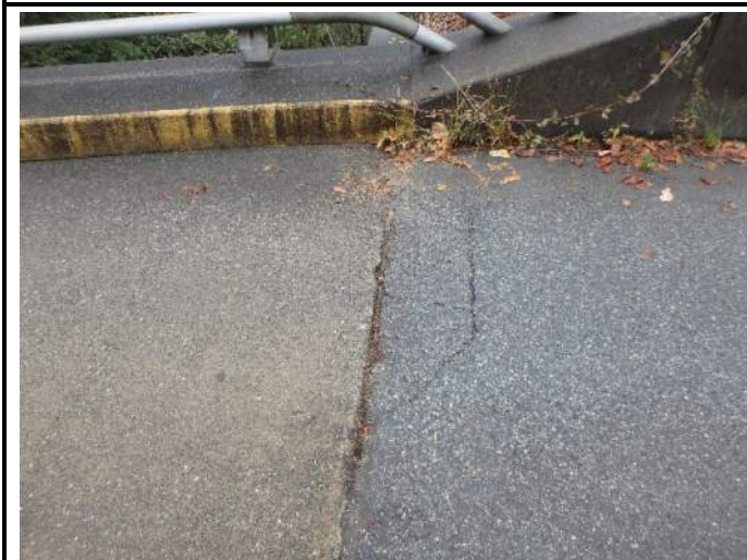
003 – Cracks at North Approach
