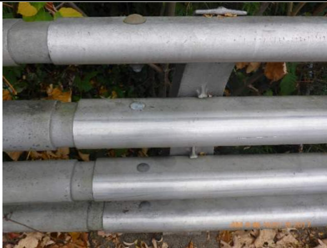
009 – Typical Railing with minor corrosion on top bolts
