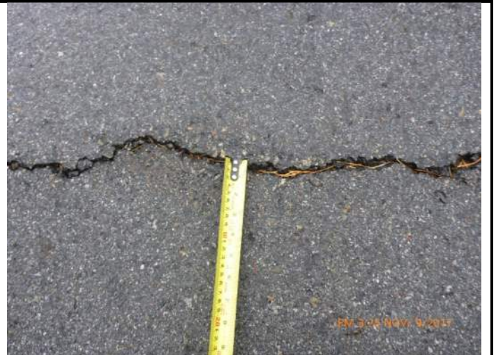
004 – Typical asphalt crack at joints
