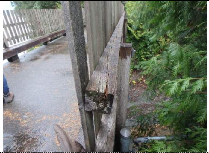
008 – Significant splits/checks, signs of decay at horizontal rails
