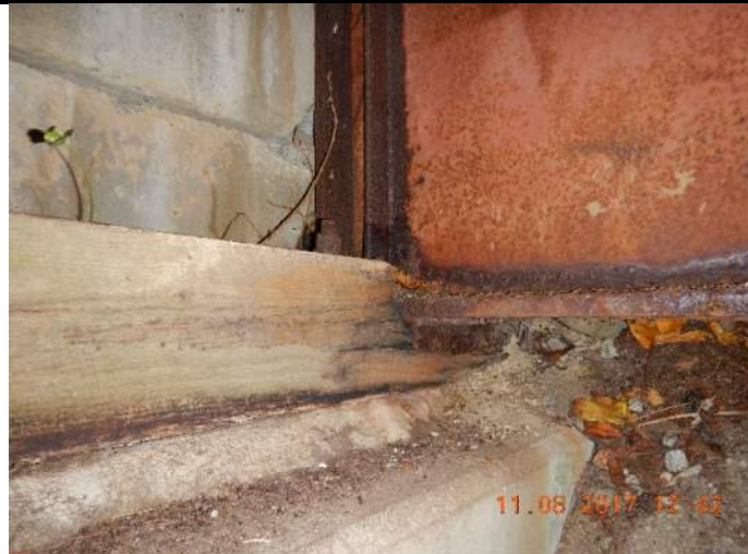
014 – Bearing at North Abutment. Note severe crushing.
