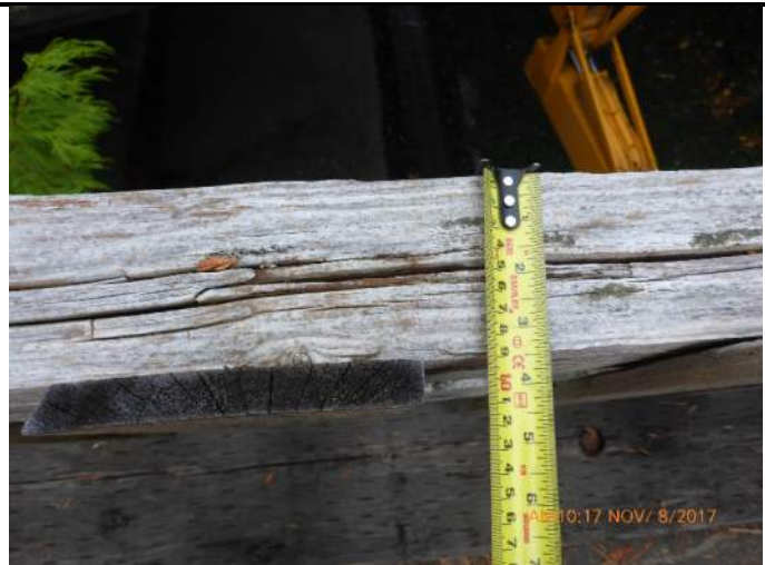
004 – Typical Railing condition – significant checks, signs of decay
