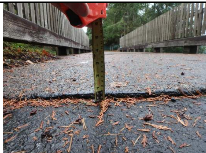
004 – 15mm difference in elevation between deck and asphalt at North approach
