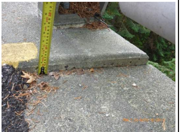
012 – Misalignment of deck and retaining wall North of bridge at West side
