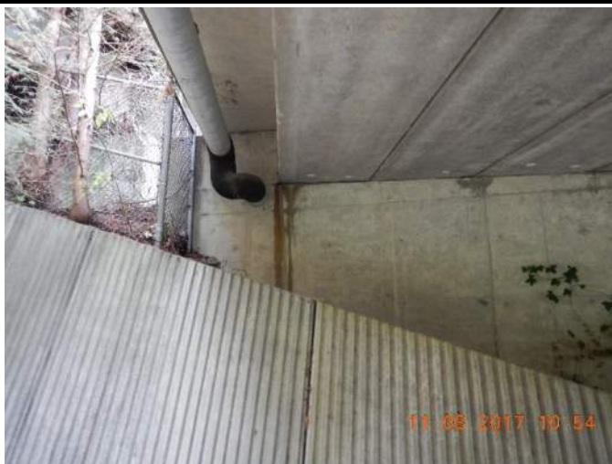
011 – South Abutment: evidence of leaking at East side
