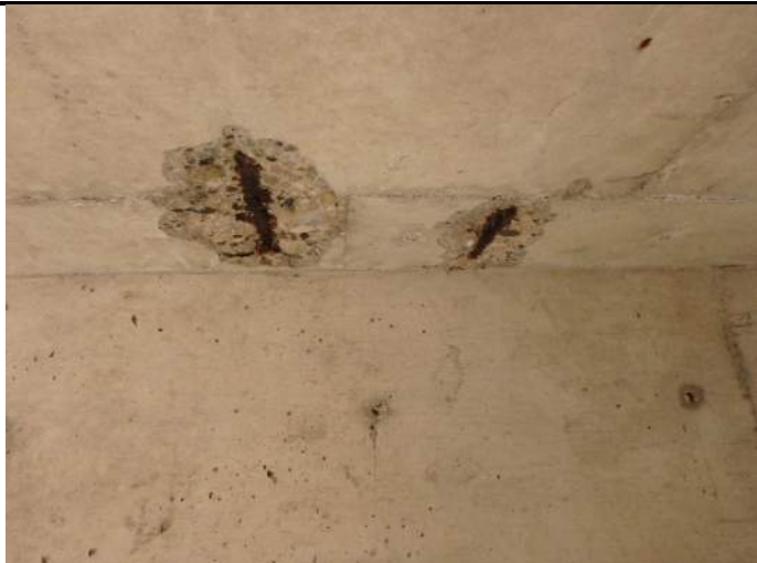
012 – Spalling with exposed corroded reinforcing on soffit, typical
