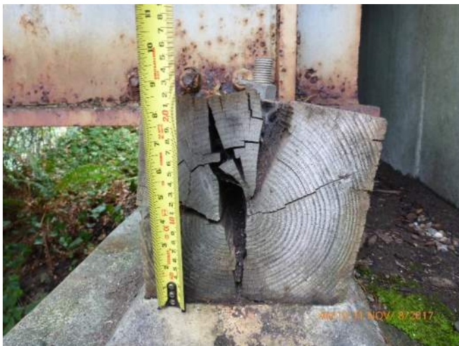
011 – Bearing at South Abutment. Note severe cracks and crushing.
