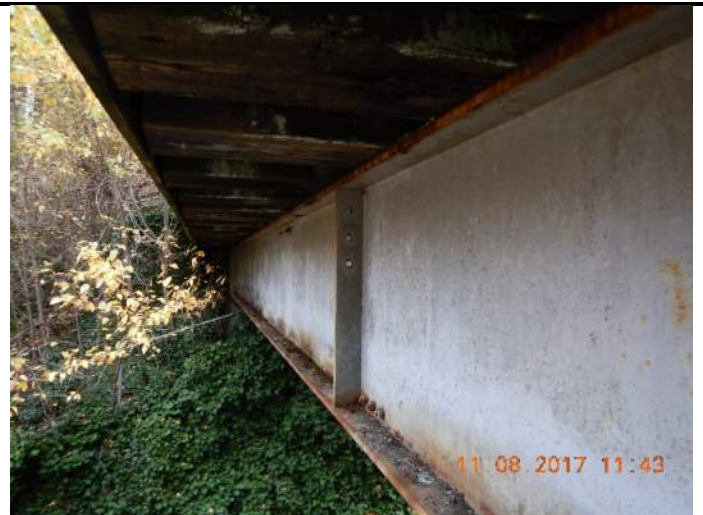
020 – Girder Exterior typical. Note surface rusting through coating.
