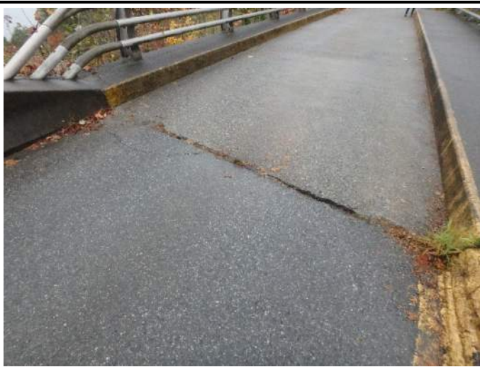
003 – South Approach – Gap between deck and approach
