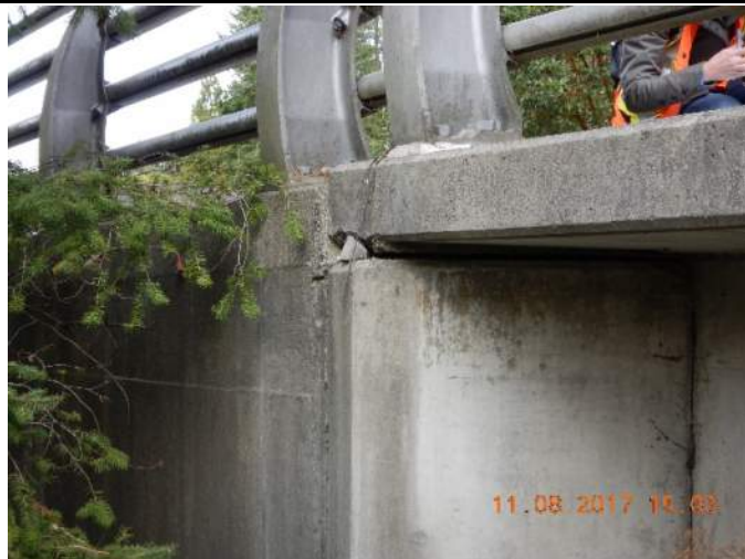
029 – North corner of West sidewalk – minor spall
