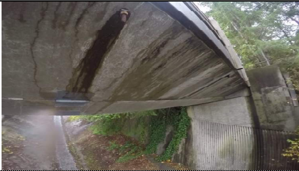
012 - Soffit overview, leakage through the bolts (hold down wheel guard)
