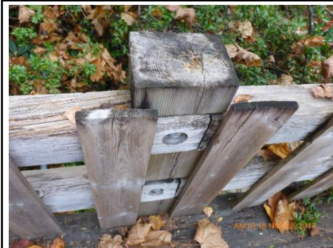
005 – Typical Post: soft timber, splits
