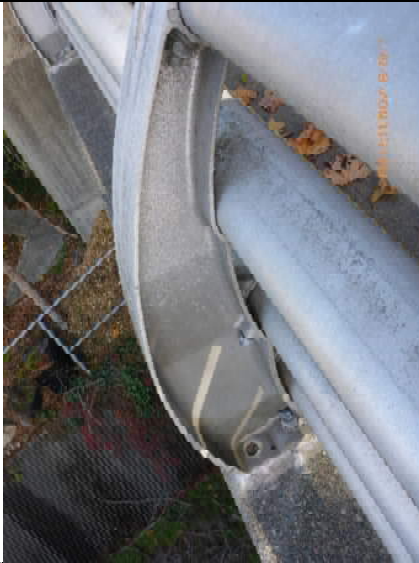
009 – Missing anchor bolt at 3 rd post from North on West side
