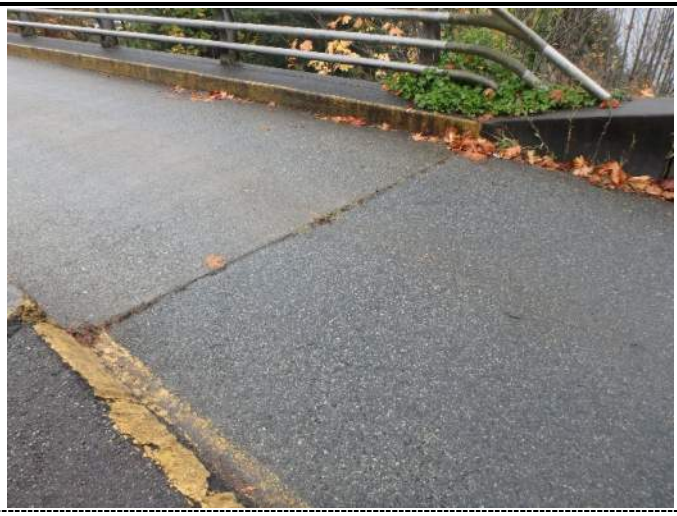
005 – North Approach – Gap between deck and approach
