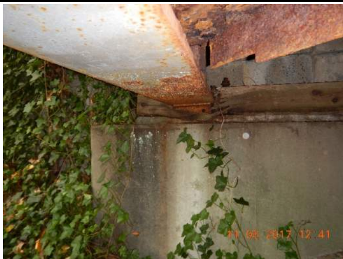
013 – North Abutment Bearing. Note severe crushing.
