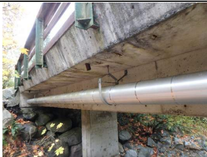
009 – Watermain on East side; spalling and exposed reinforcement bars typical throughout
