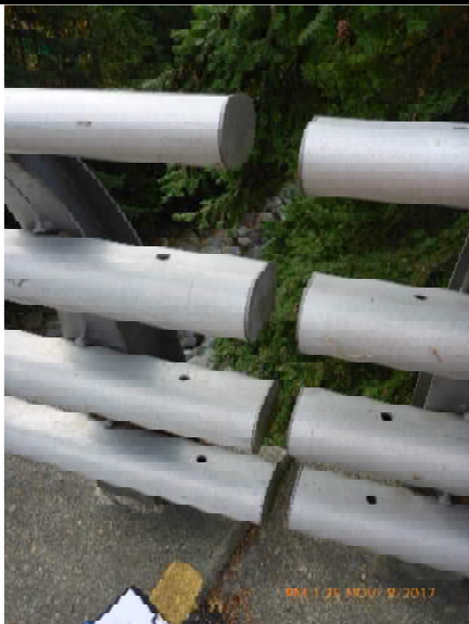
011 – Misalignment of railings at North-West corner
