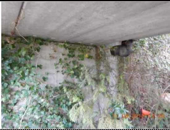
013 – Leaking at exterior girder units at North Abutment
