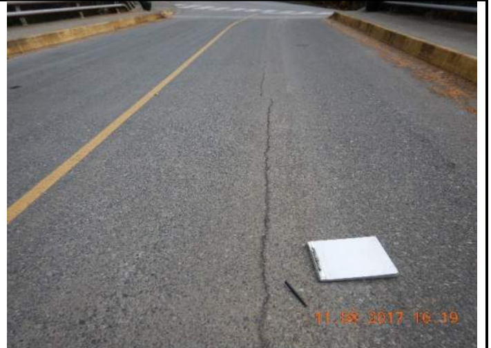
016 – Longitudinal crack at SB lane
