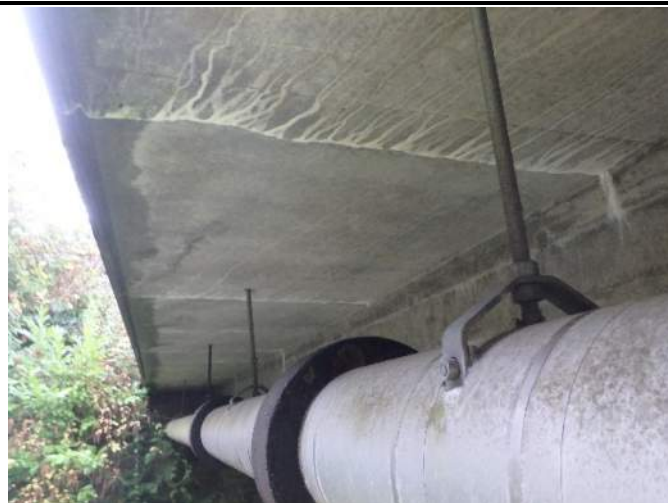
015 – Transverse cracks with efflorescence on the underside of sidewalk typical
