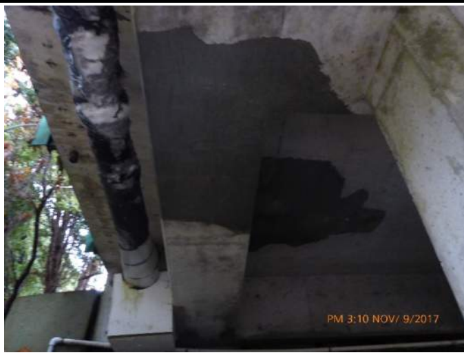
019 – Previous repairs at the soffit and Girder 2
