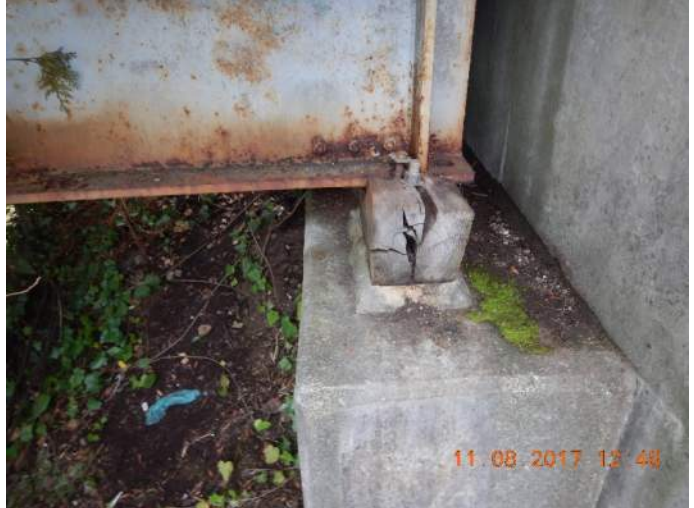
010 – South Abutment Bearing. Note severe cracks and crushing.
