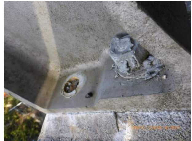
010 – Close up of missing anchor
