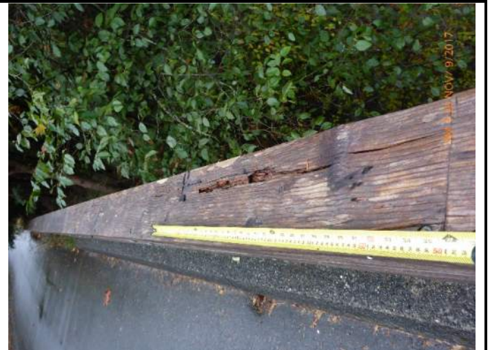
006 – Typical decay at the top rail
