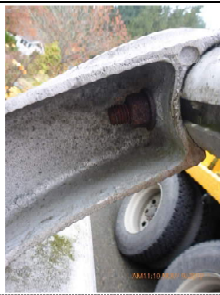
008 – Rusting bolt at the railing post
