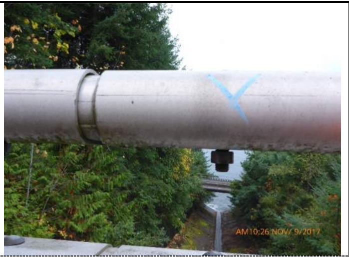
008 – Loose splice bolt at West side railing
