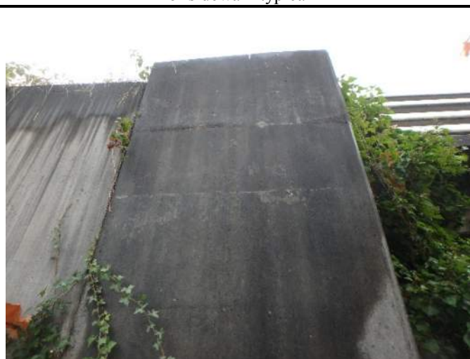
017 – Hairline cracking at North Abutment wall
