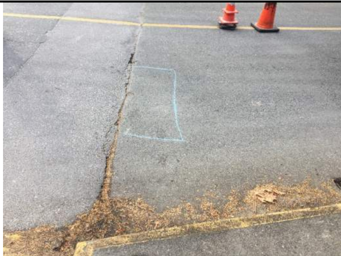
005 – Delamination area at South-East side of deck
