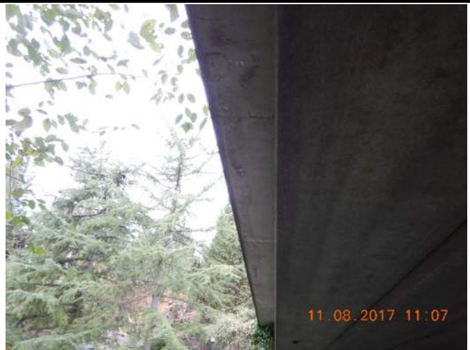
017 – Curb underside. Note transverse cracks with efflorescence.
