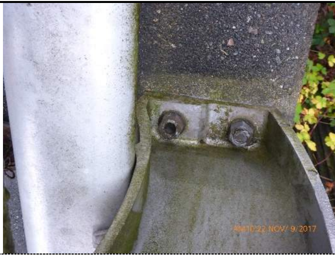
007 – Anchor bolts of insufficient length (2 locations)
