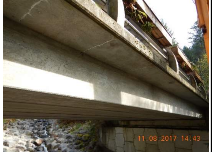
018 – Transverse cracks with efflorescence on underside of West sidewalk, similar observed at East sidewalk
