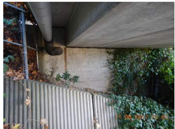
012 – Leaking at exterior girder units at South Abutment
