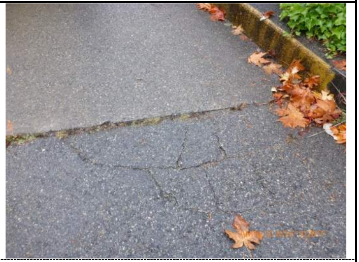
006 – Crack in asphalt at North Approach, West side
