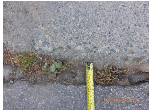
006 – Vegetation in the gap and abrasion at the deck due to uneven elevation at South Approach
