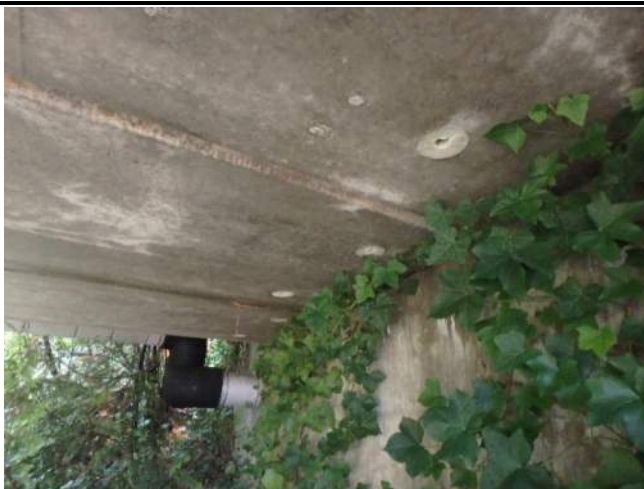
011 – Vegetation at S approach, evidence of water leaking between girders
