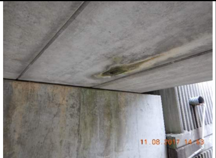
026 – Drains are flush with girders
