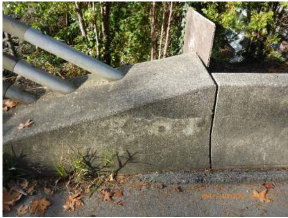
007 – Efflorescence at the curb at North-West end
