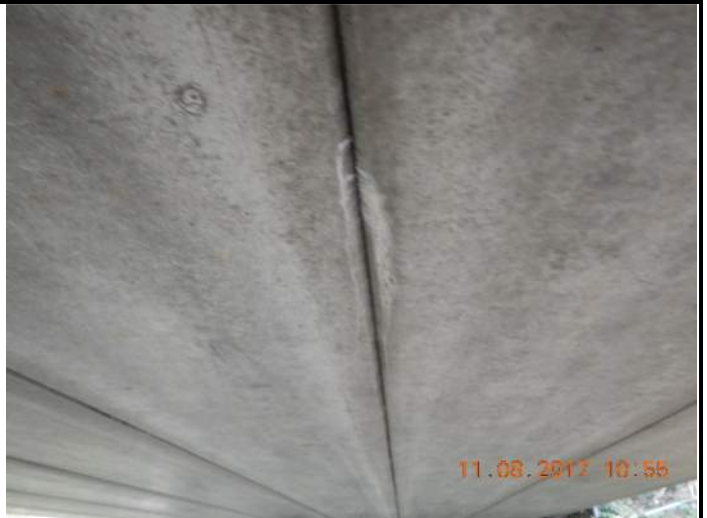
014 – Localized efflorescence between girders
