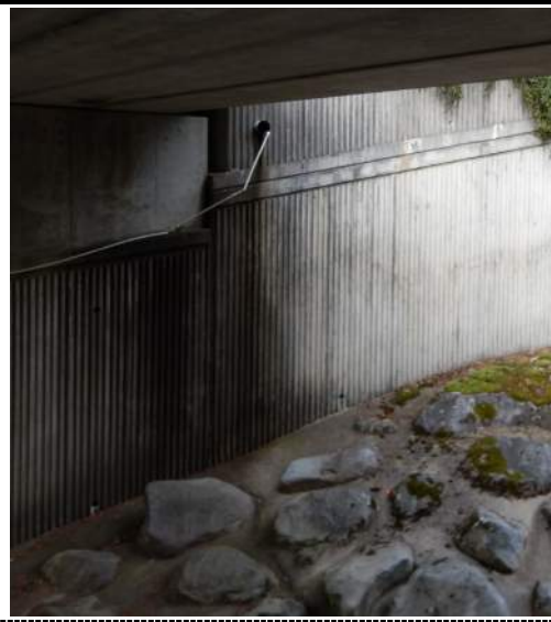
022 – Evidence of leaking at North Abutment
