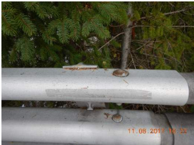
017 – Rusty bolts at railing, typical
