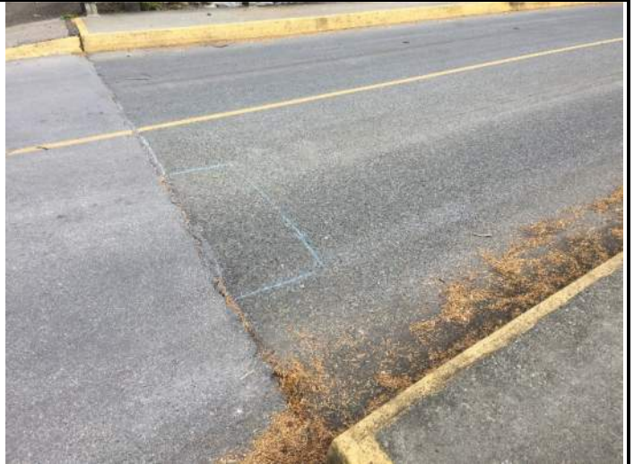
008 – Delamination area at North-West side of deck
