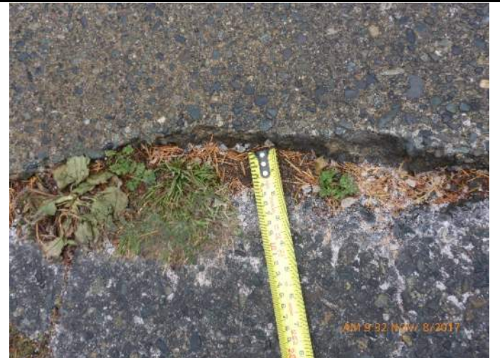
004 – Gap between deck and asphalt at South Approach
