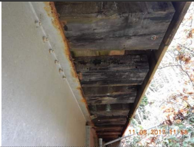
021 – Suspected rotting at floor beams
