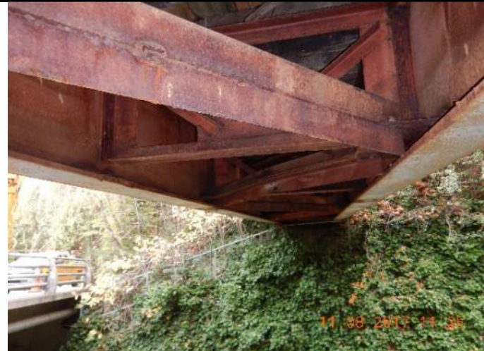
018 – Medium corrosion on all bracing/diaphragm members
