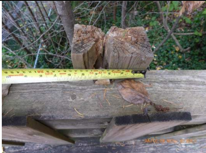
006 – 8 posts are failing (significant crushing)
