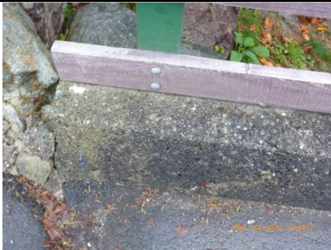
005 – 0.8m long delamination at North end of East side curb
