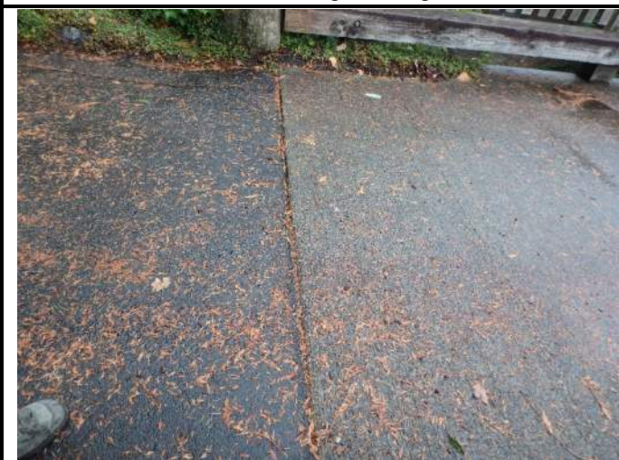
003 – Minor gap between deck and asphalt at South approach
