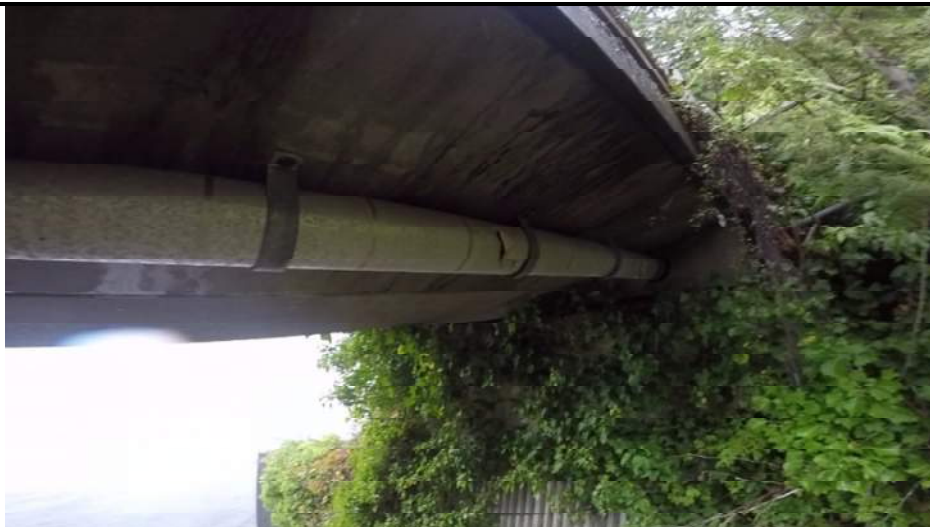
010 – North Abutment Overview – vegetation overgrowth; water main on the East side of the bridge
