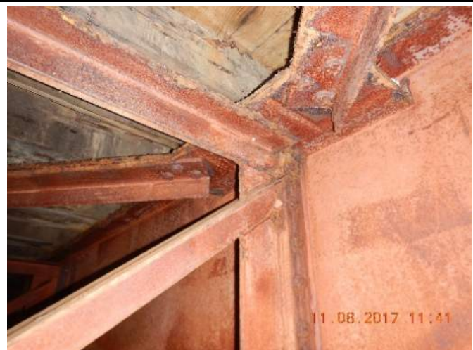
017 – Typical Connection – medium corrosion
