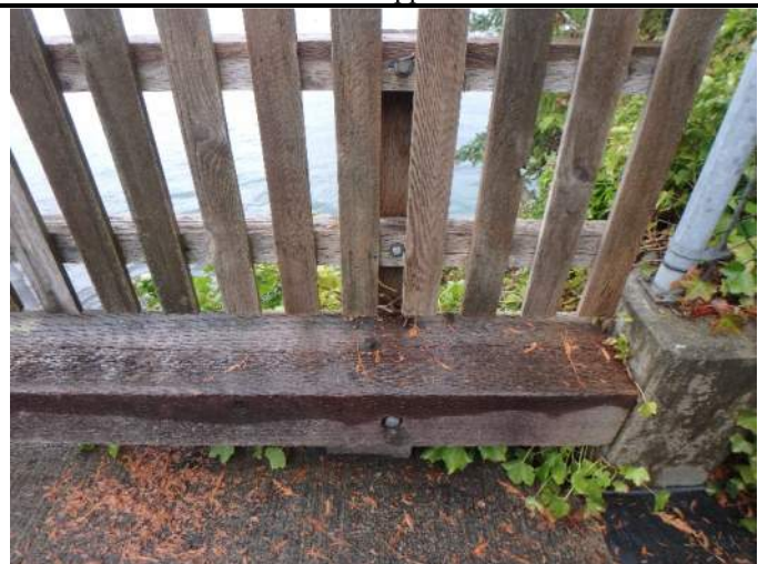
006 – Vertical plans in fair condition, all connections are poor (not adequate for load)
