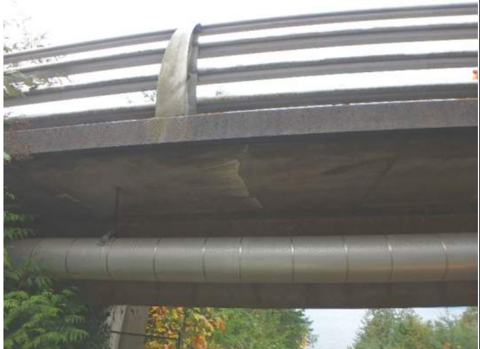
012 – Typical transverse cracks with efflorescence at the underside of sidewalks
