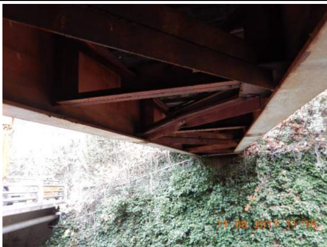
015 – Girders and diaphragms overview – medium corrosion on flanges and light corrosion on web. Note permanent deformation on cross bracing.
