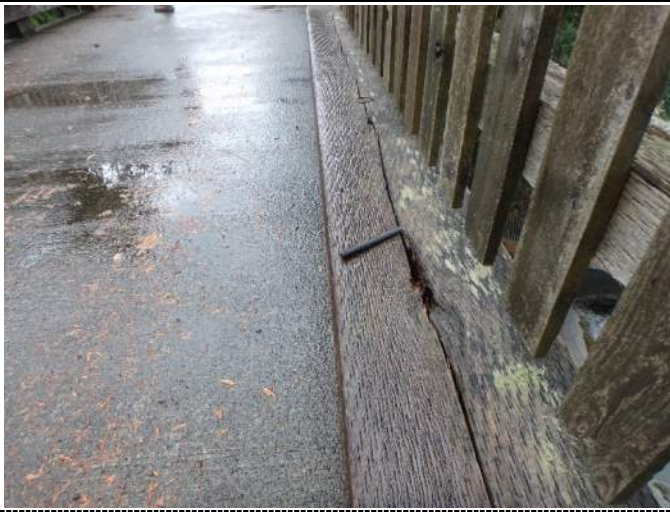
007 – Deep splits/checks, rot throughout wheel guard
