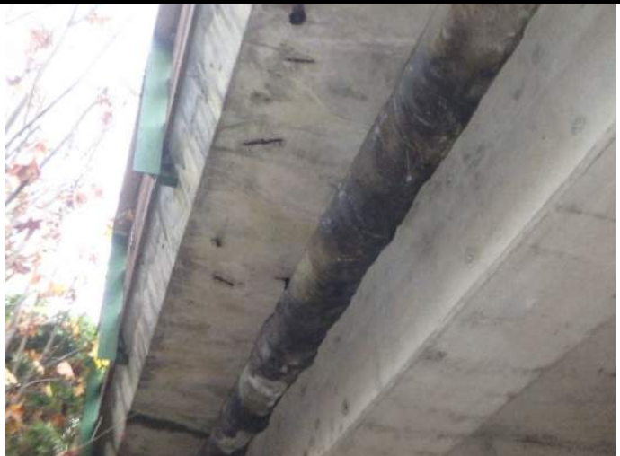
016 – Main at West side, typical exposed rebars
