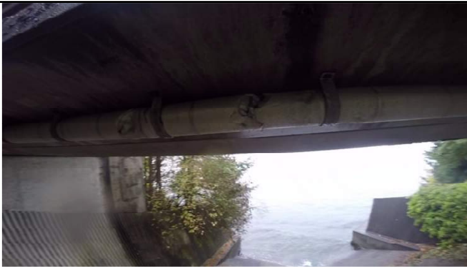
011 – Water main is damaged in several sections
