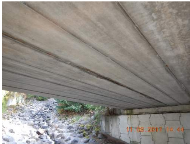
027 – Leaking through Girders 5 and 6 with efflorescence
