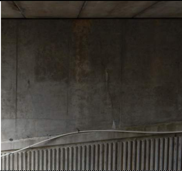
021 – North Abutment: vertical hairline crack with efflorescence, localized rust staining
