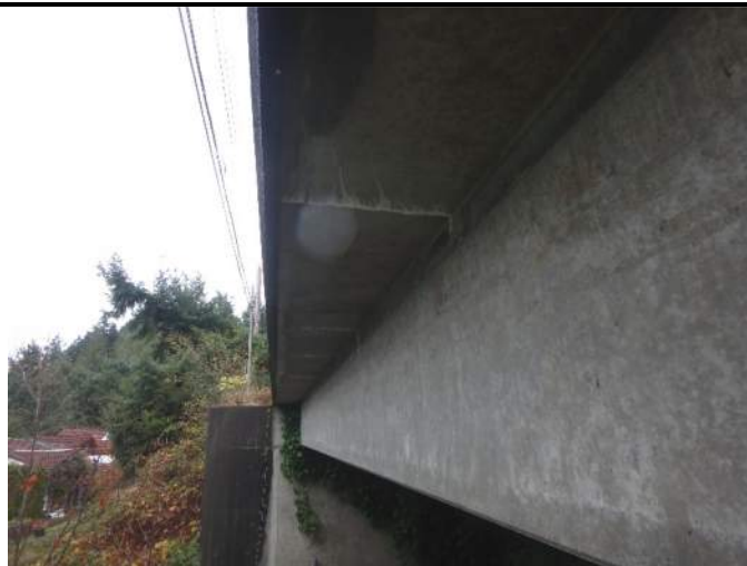
014 – Transverse cracks with efflorescence at the underside of curb typical.
