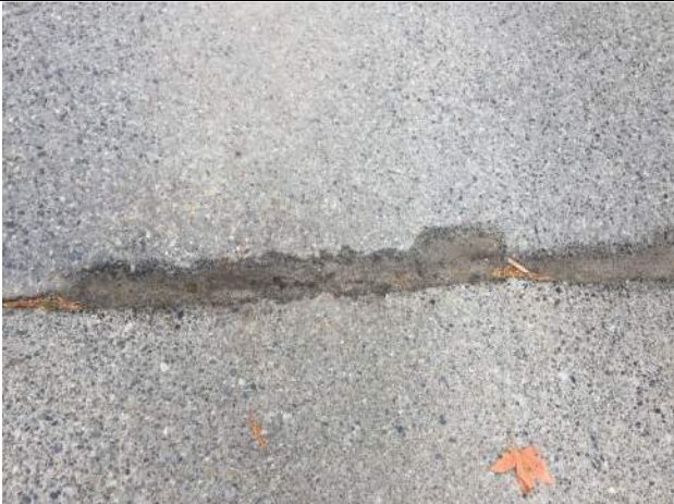
003 – Gaps between deck and asphalt at North Approach
