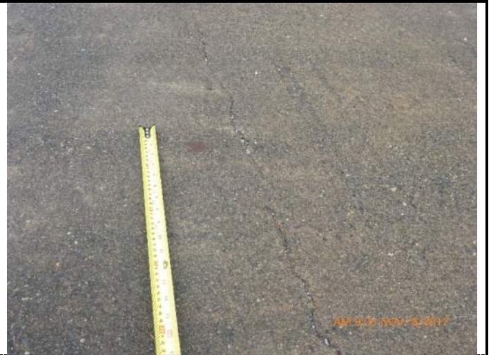
008 – Hairline crack at SB lane on Deck
