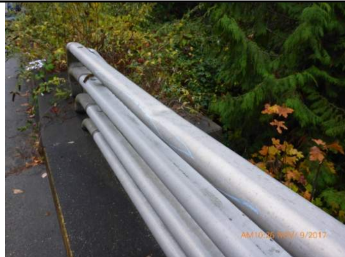
006 – Deformed rail on West side
