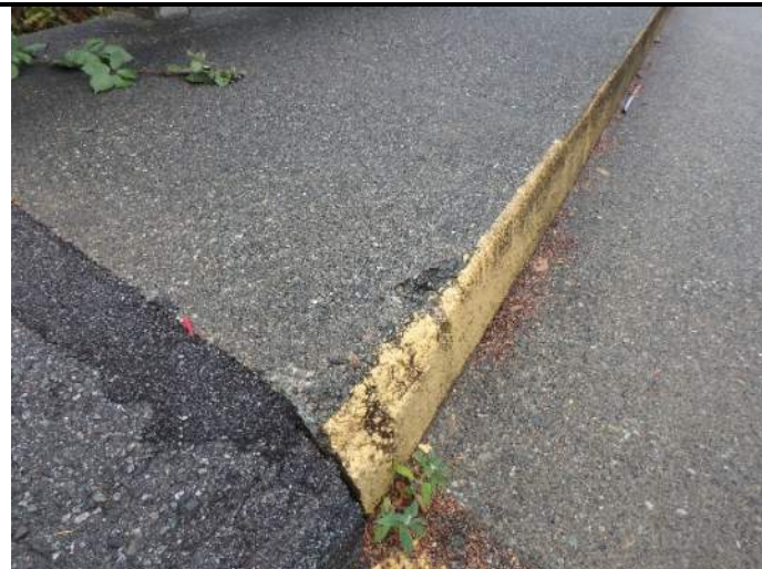
004 – Minor spall at sidewalk edge on North side
