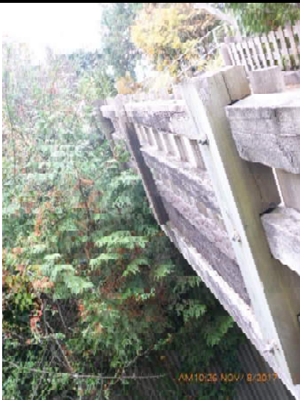
007 – Typical Post connection to wheelguard
