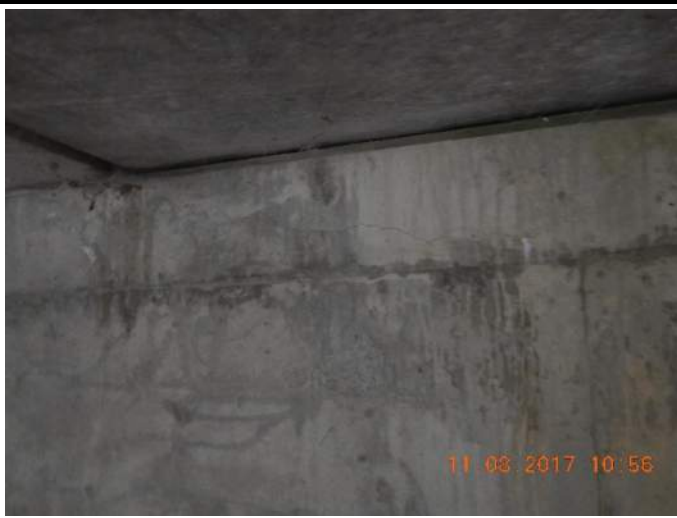
013 – South Abutment: medium hairline crack under Girder 4
