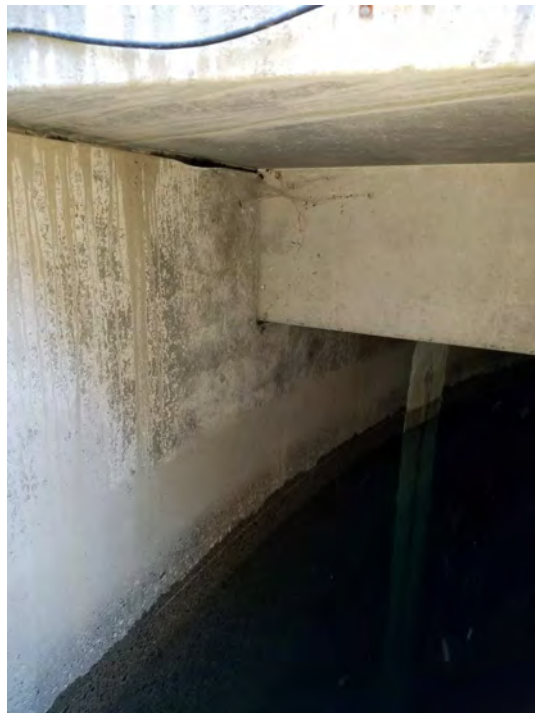
Figure A2.3.4: Roof support beam observed from access hatch opening
