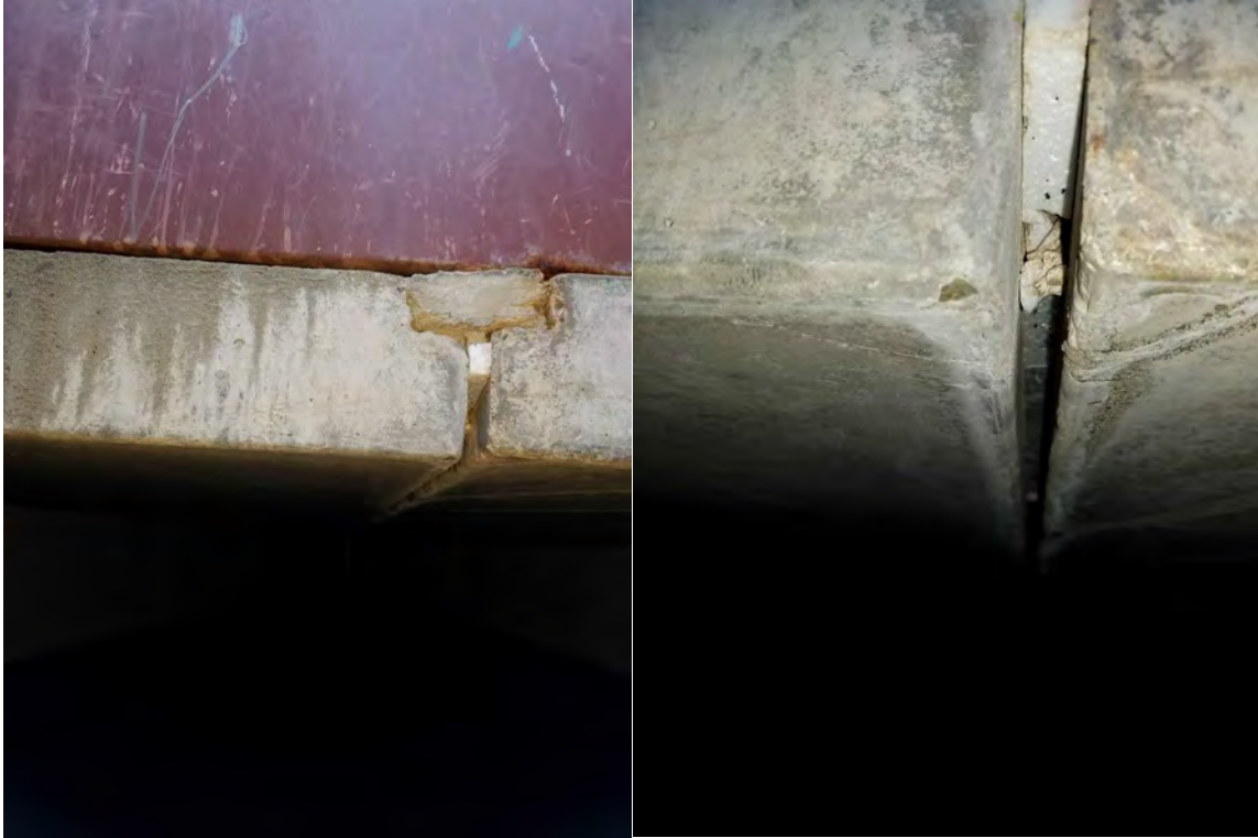
Figure A2.3.3: Roof panel joint cross-section observed at access hatch opening
