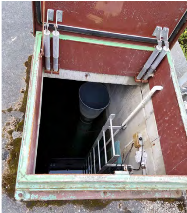
Figure A2.3.1: Roof access hatch
