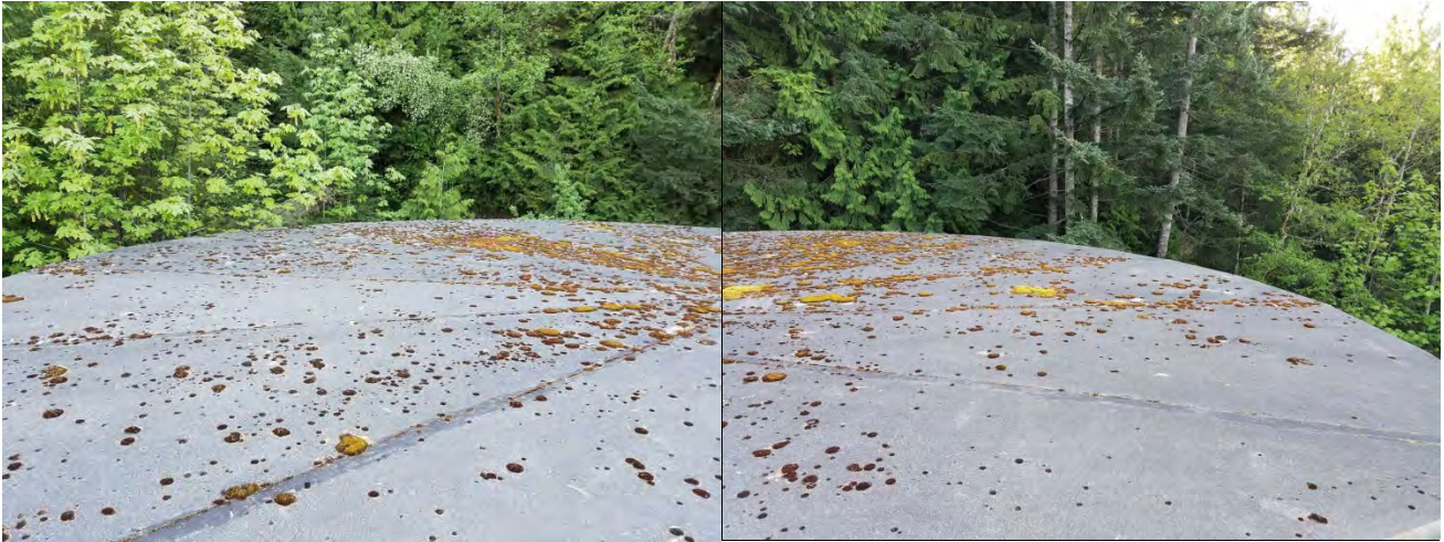
Figure A2.2.1: Roof facing southeast (two photos)
