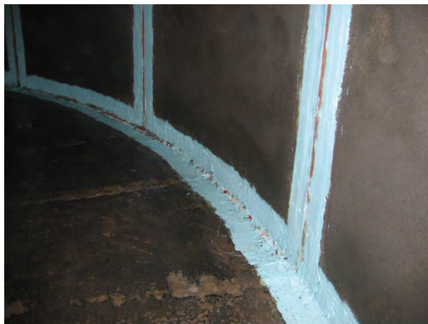
Figure 2: Record Photo of Internal Tank Joint Sealant (Feb 27, 2006)
