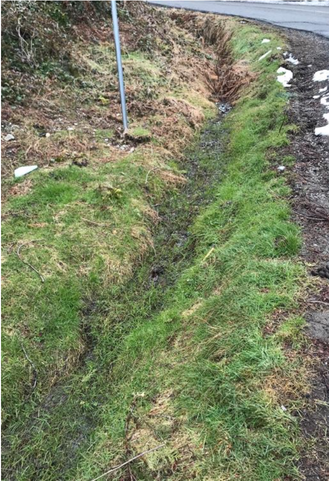
The not bedded trench on east side of Oceanview Road, down from 245
