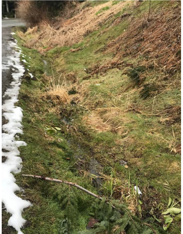
The not bedded trench on east side of Oceanview Road, down from 245
