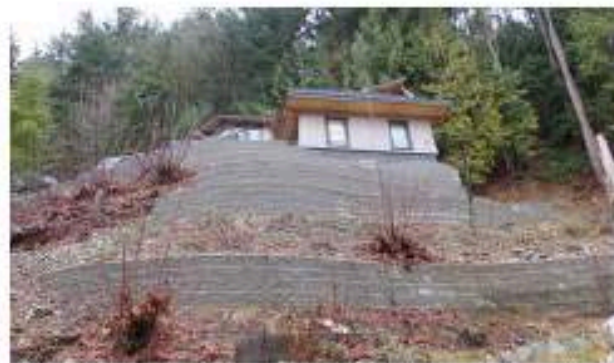
Many homes situated on steep slopes require extensive retaining systems.
