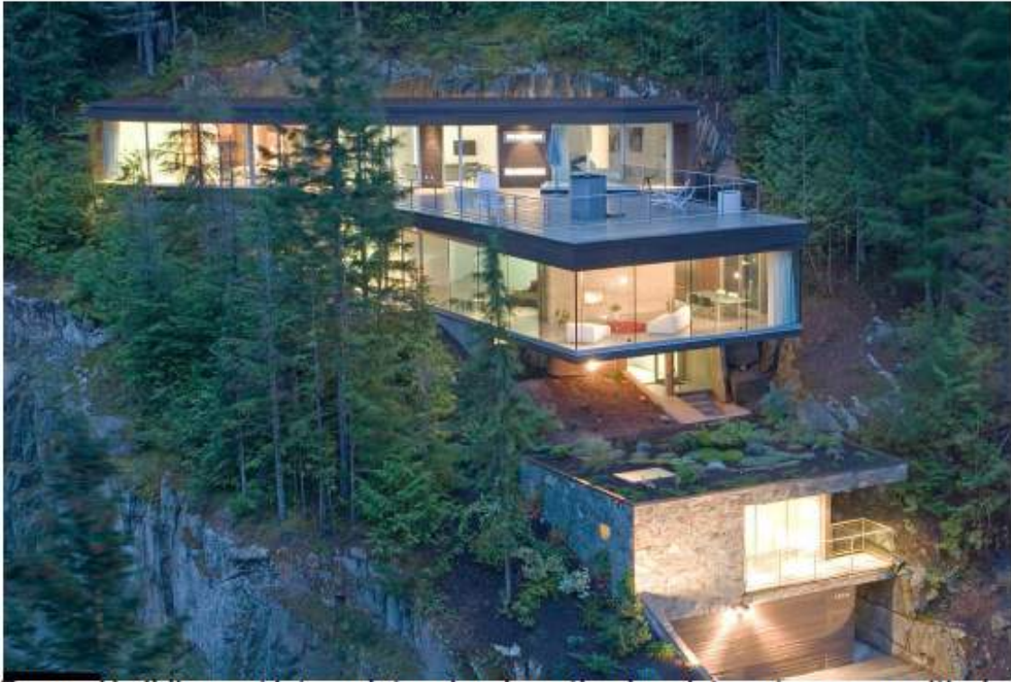
Terraced buildings set into and stepping down the slope Integrate more sensitively into the steep hillside environment
