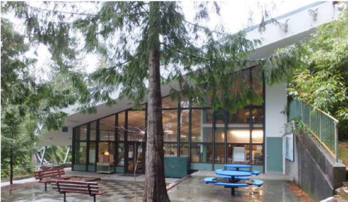
The Village School is a good local example of a terraced building set sensitively into its context
