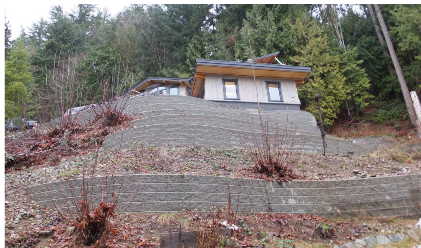
Many homes are situated on steep slopes and require extensive retaining systems.
