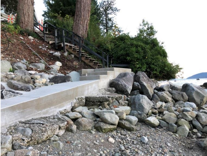
Figure #5: Beach Obstruction with Boulders/Rock
