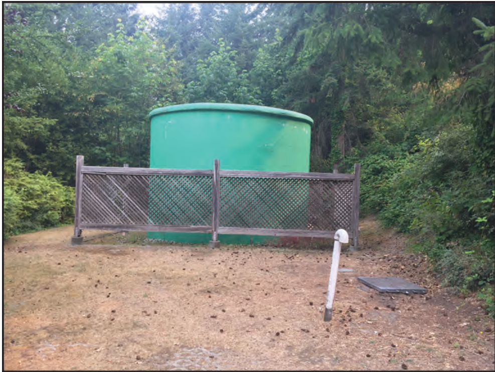
Figure 24: Highway Tank, facing north.
