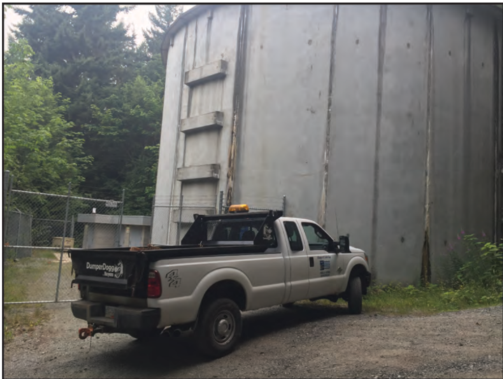
Figure 19: Harvey Tank, facing north by northwest.
