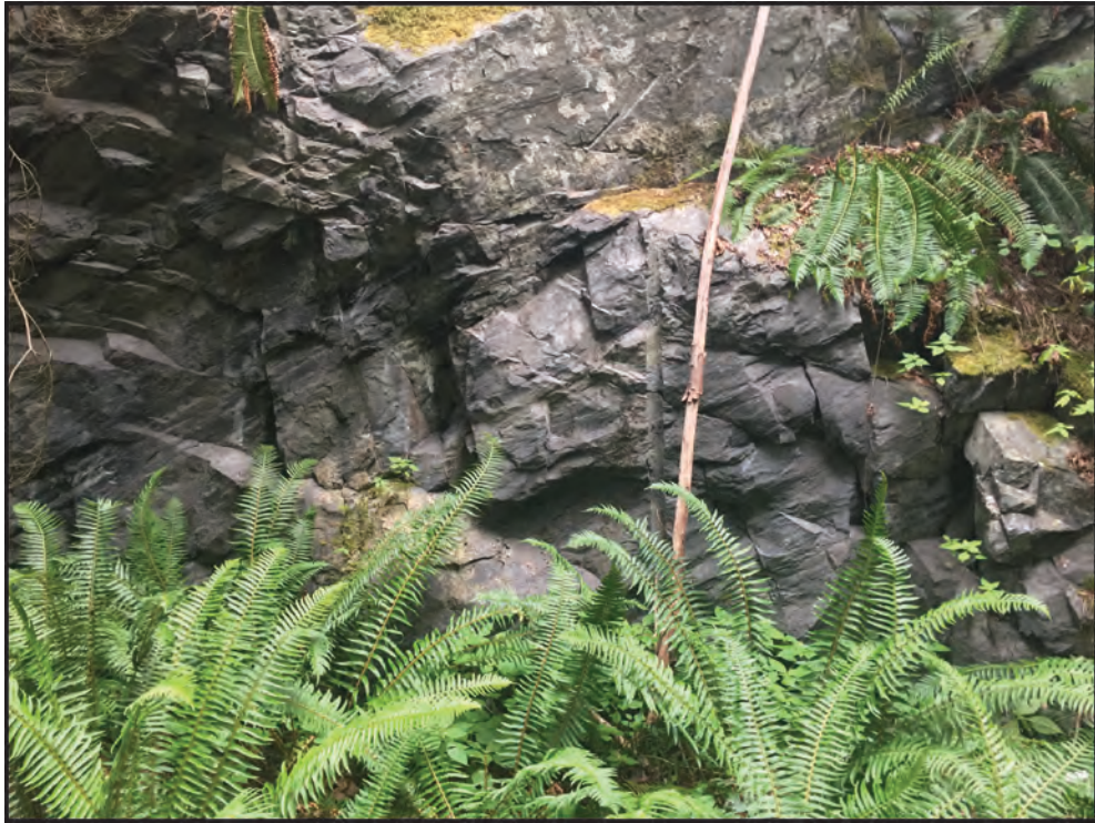
Figure 23: Basalt exposure behind Harvey Tank. Blasting tube visible in middle of photograph, facing east.
