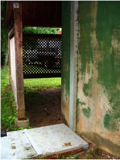
40. Fill station sensing line
