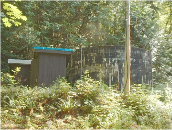
82. General view of tank
