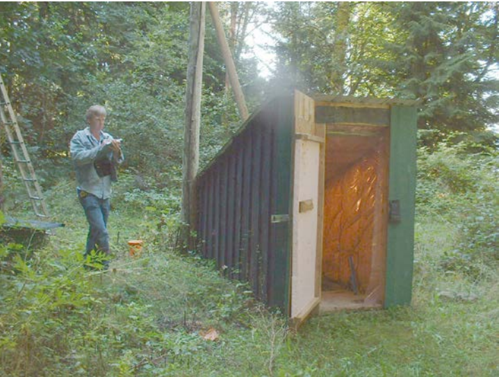
80. General view of valve chamber
