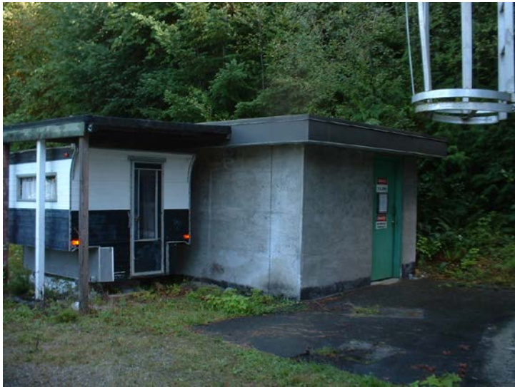
63. General view of chlorination building
