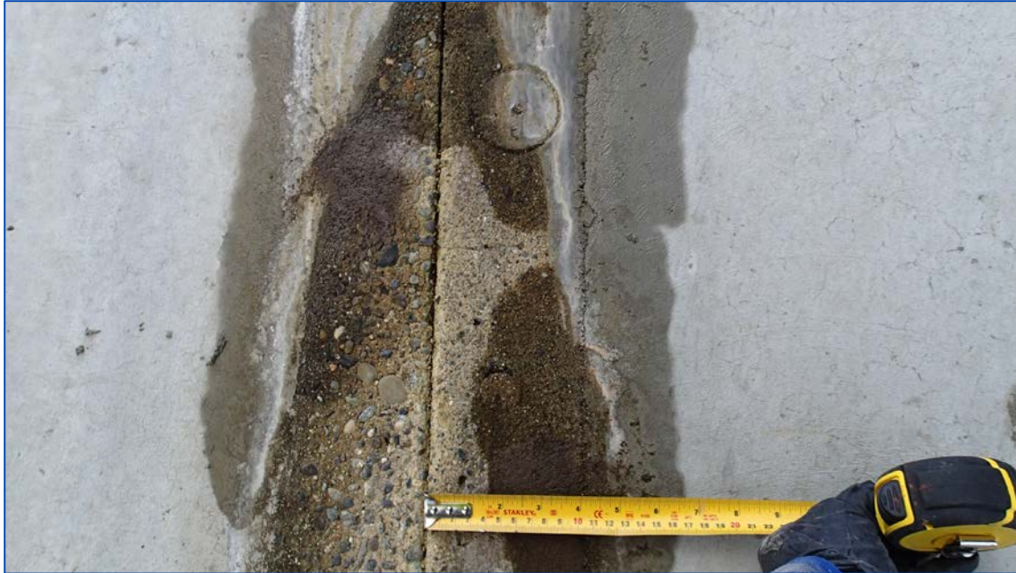
Photo 3: Infilled concrete strip at the joint between the precast wall panels.
