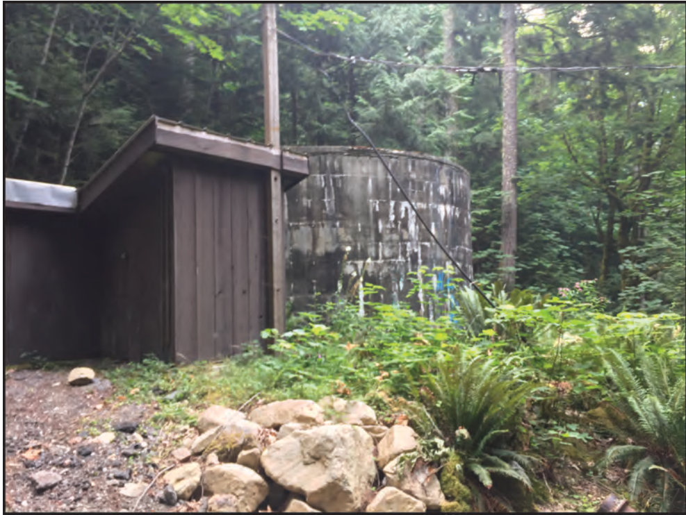
Figure 18: Phase V Tank, facing south by southeast.
