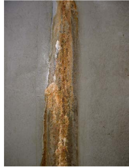
50. Leak at panel junction showing possible corrosion staining
