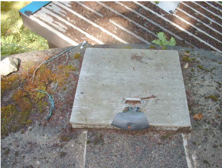
88. View of hatch on roof
