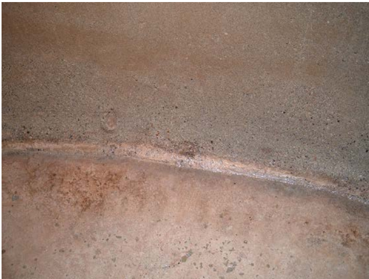
173. Joint between reservoir interior wall and floor in good condition
