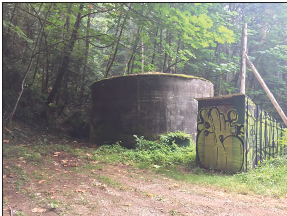
Figure 11: Phase IV Tank, facing southeast.
