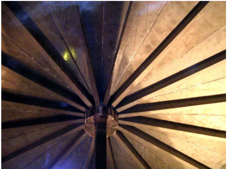
142. Underside of roof from inside of tank
