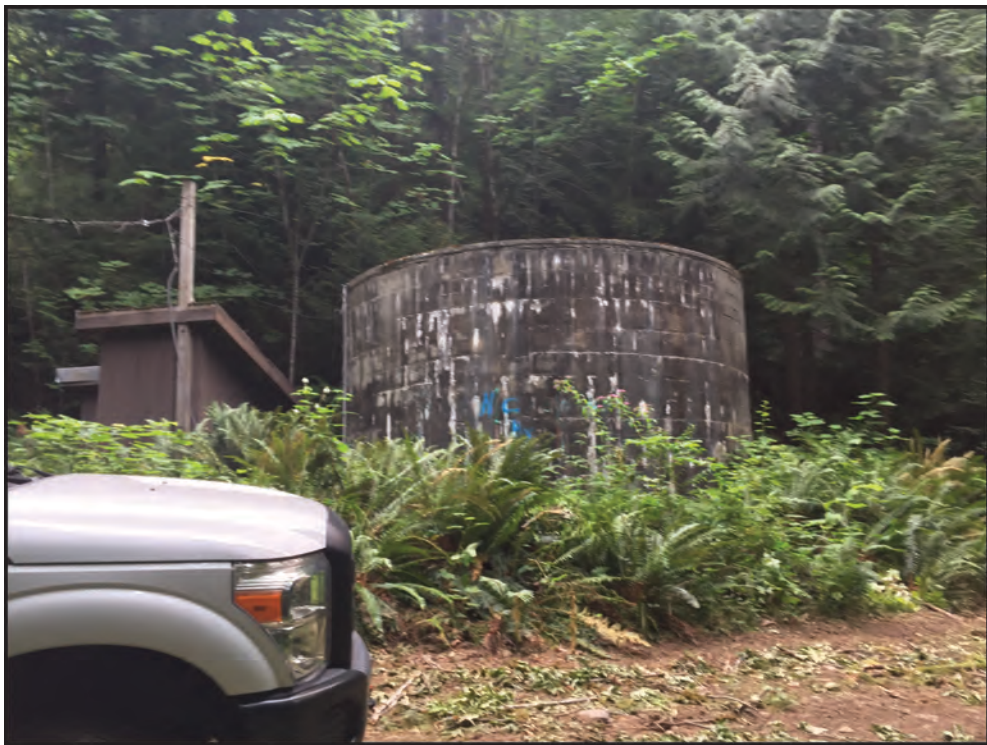
Figure 17: Phase V Tank, facing east.
