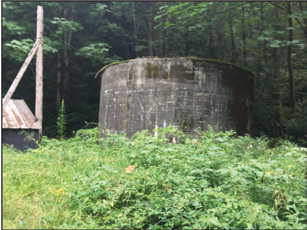
Figure 12: Phase IV Tank, facing north by northeast.
