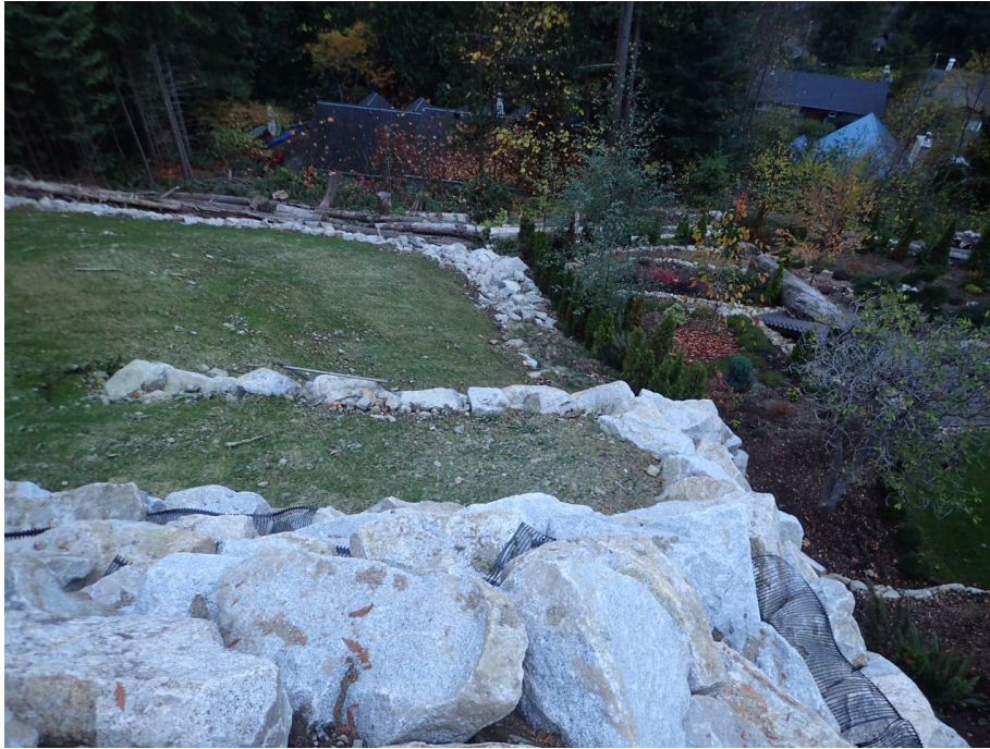
Photo 15. Stacked rock wall in steep terrain using geotextile to tie back into slope.
