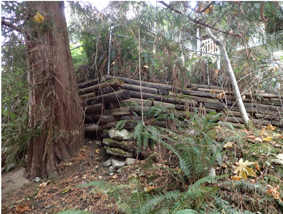
Photo 16. Substandard retaining walls represent a slope hazard.
