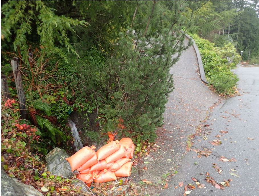
Photo 7. Lot 66 Kelvin Grove Way. Small Creek captured by drainage system undersized for full range of flows requires sand bagging to prevent overflow onto local road.
