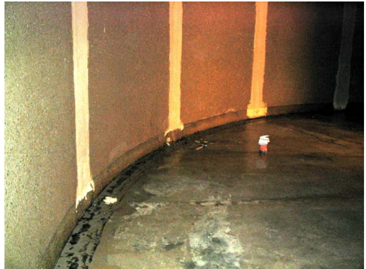
148. Rubberized type of coating material used along joint between the wall and base slab
