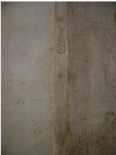
53. "Closing in" section of concrete between two wall panels at North side of tanks
