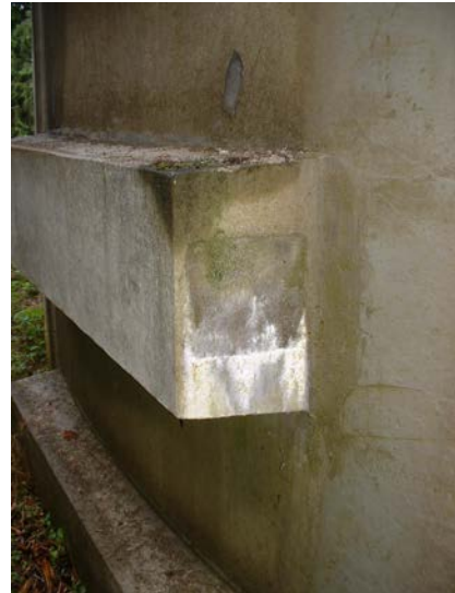
52. Note efflorescence at SE anchor block
