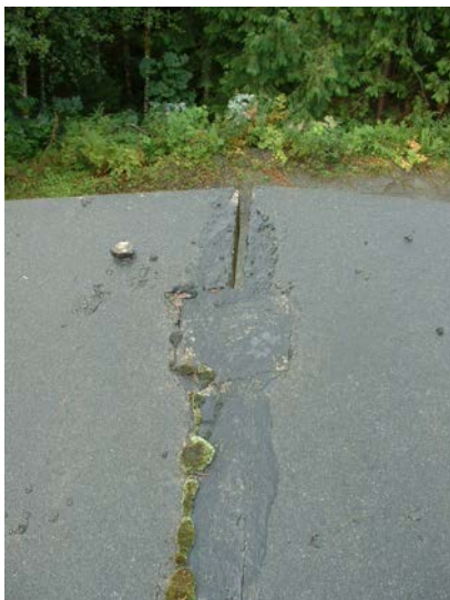
59. Concrete filler section has fallen out from between two precast concrete roof panels
