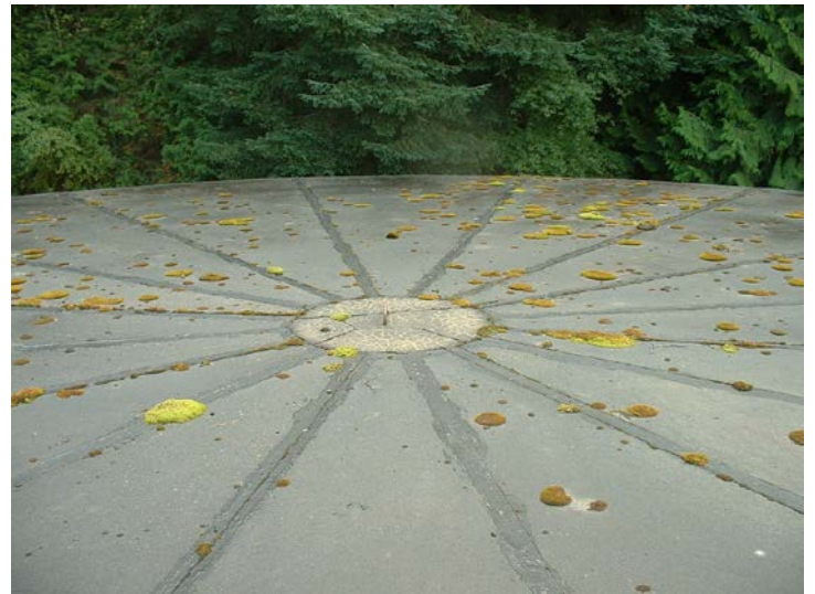
58. Note concrete precast panels making up the roof structure
