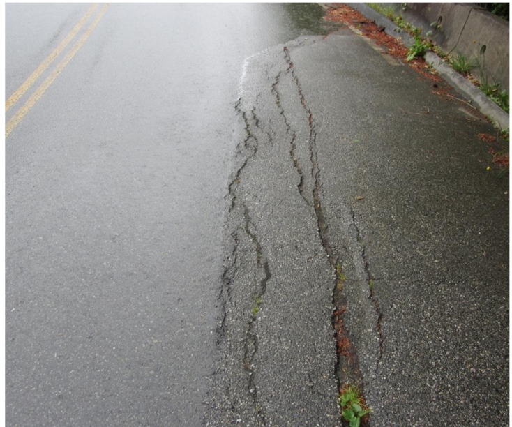
Figure 5-2: Photo of Edge Cracking
