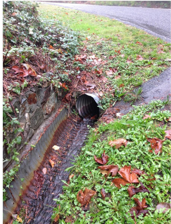
Figure 4-2: Photo of Corrugated Steel Pipe Culverts
