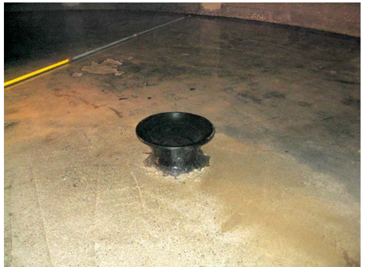
144. 250 Φ bellmouth inlet drain
