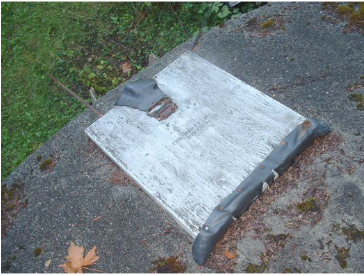
78. Roof access hatch
