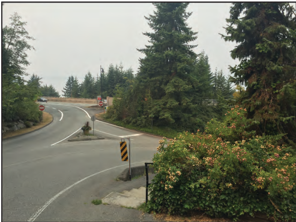
Figure 26: Looking out from the entrance to the Highway Tank location toward Highway 99, facing west.
