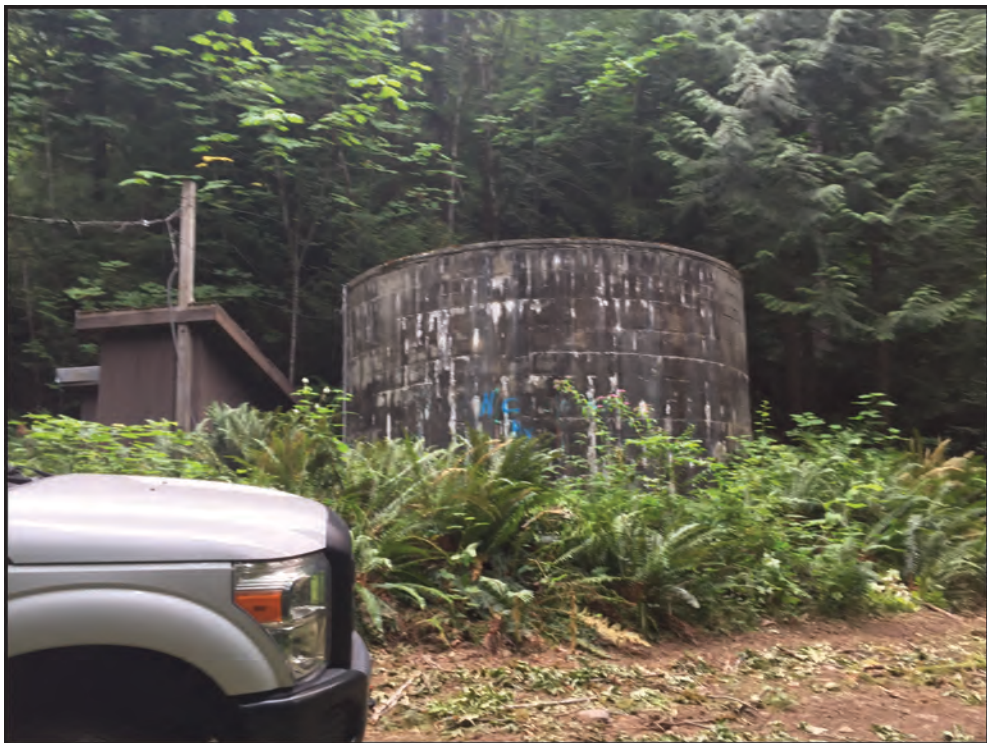
Figure 17: Phase V Tank, facing east.
