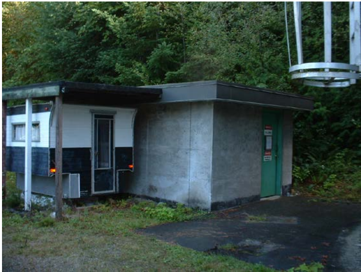
63. General view of chlorination building
