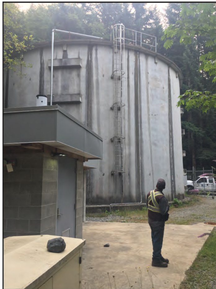
Figure 21: Harvey Tank, facing southeast. Darrell Guss in foreground.
