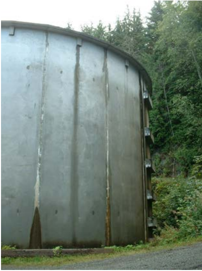
49. Eastern side of tank showing east side anchor blocks and further leaks
