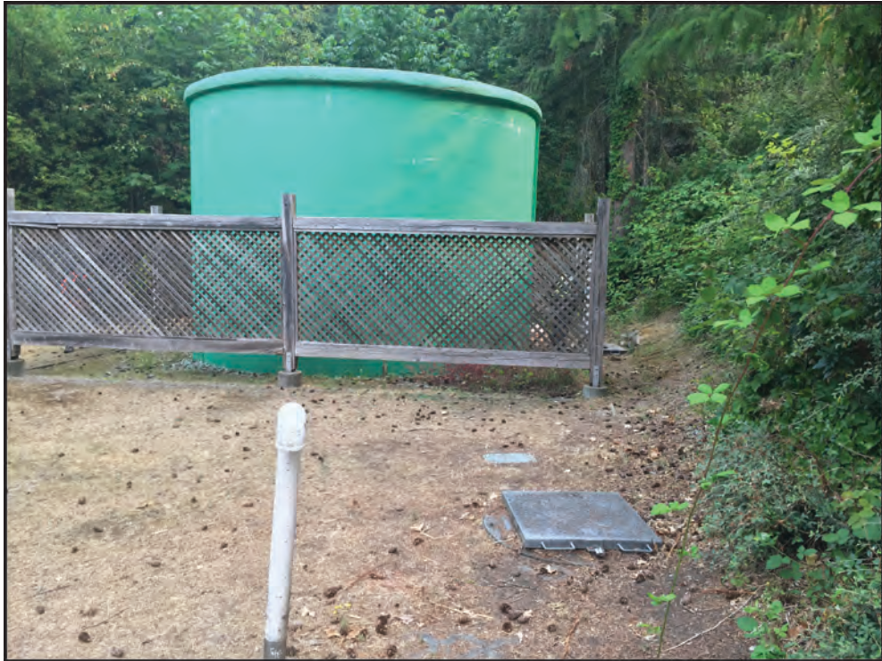
Figure 25: Highway Tank, facing north.
