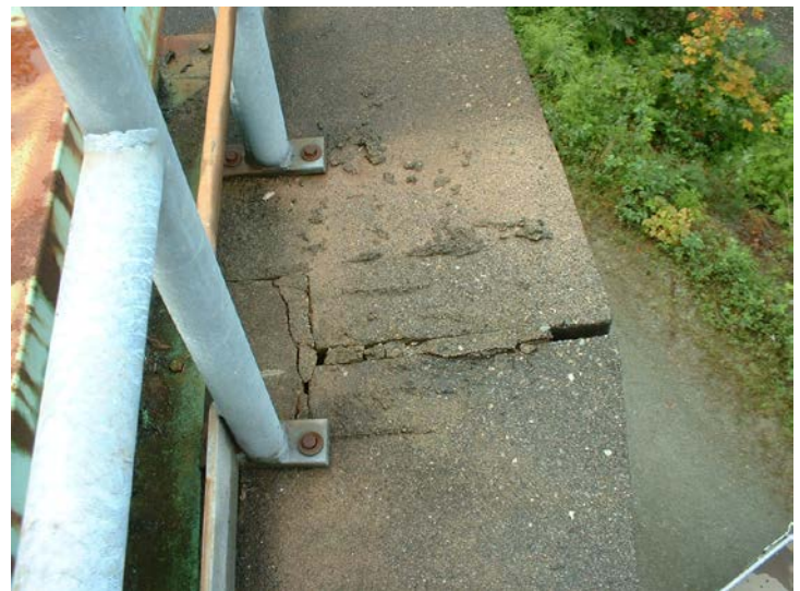
60. Joint between precast concrete roof panels at access hatch
