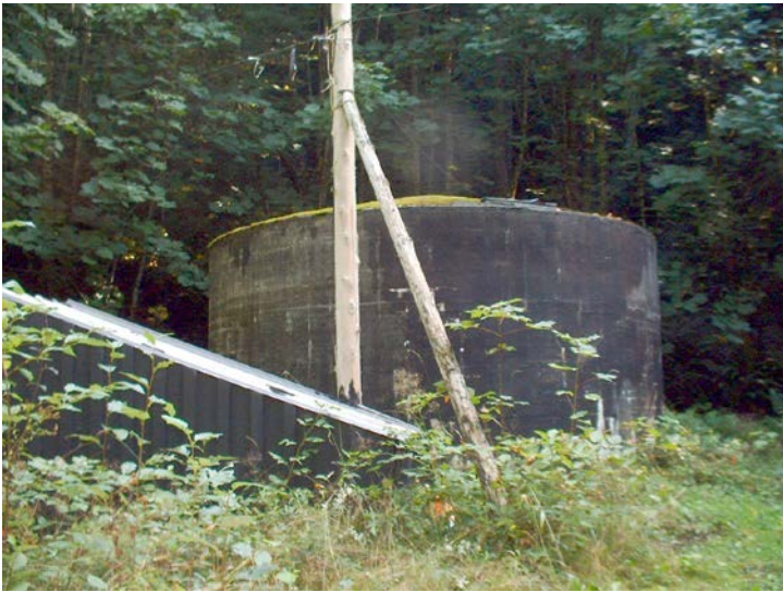
71. General view of tank
