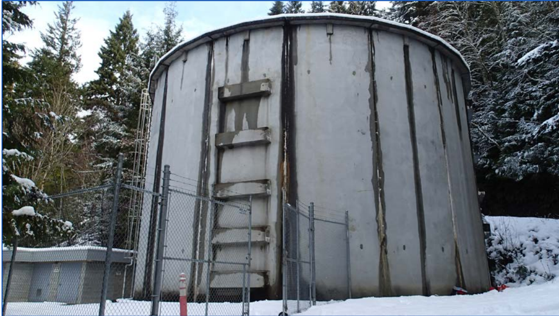
Photo1: General view of the Harvey Creek Reservoir.
