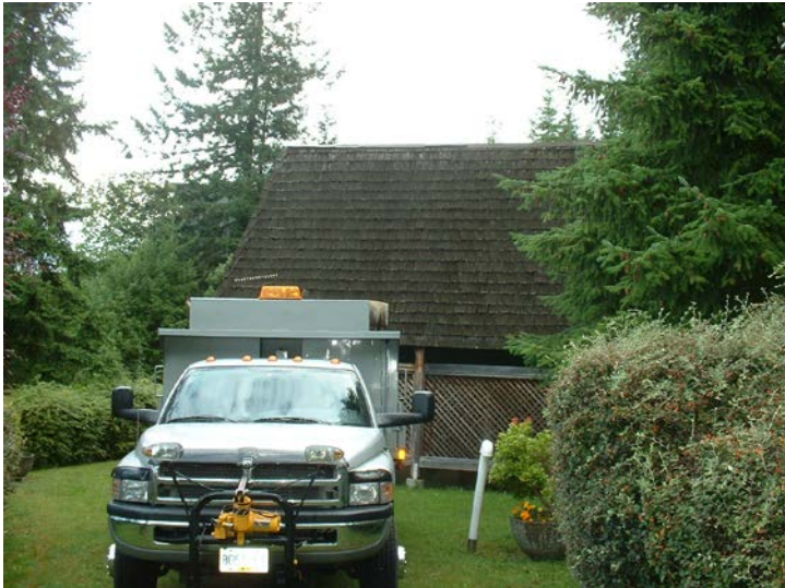
35. General view of roof structure
