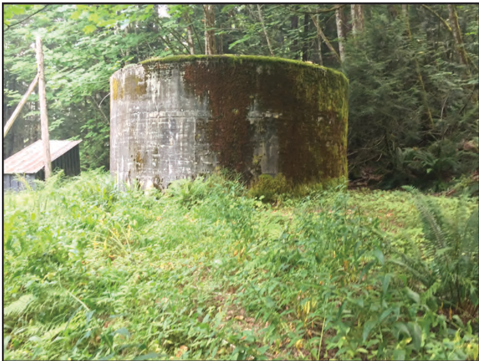
Figure 13: Phase IV Tank, facing north.
