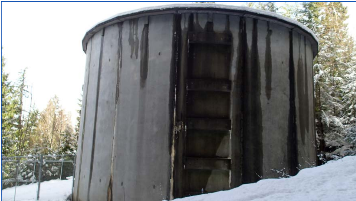
Photo 2: General view of the Harvey Creek Reservoir.
