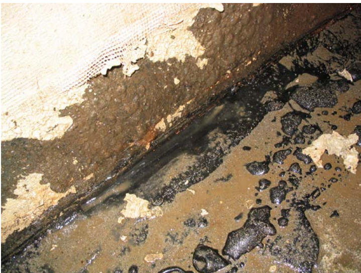
149. Evidence of failure (note air or water bubbles visible on the surface of the material) in the sealing material along joint between wall and base slab.
