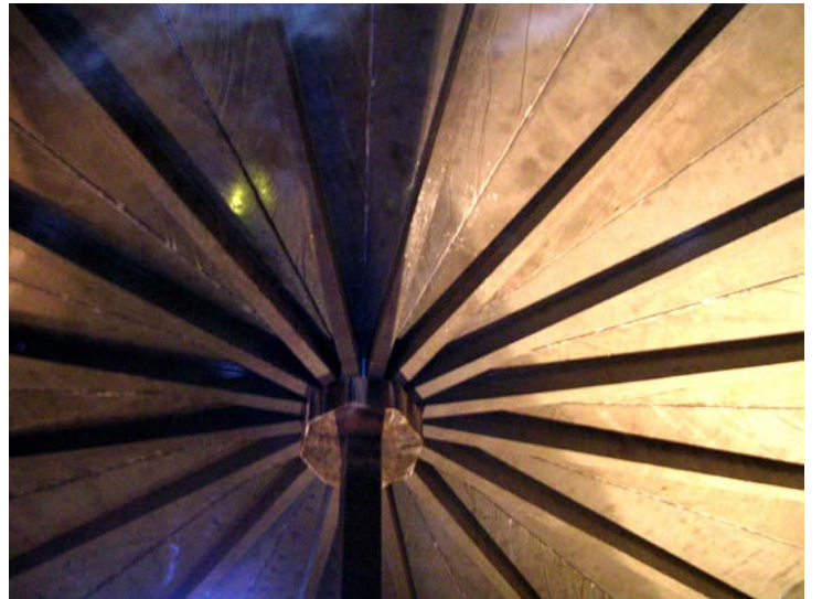
142. Underside of roof from inside of tank
