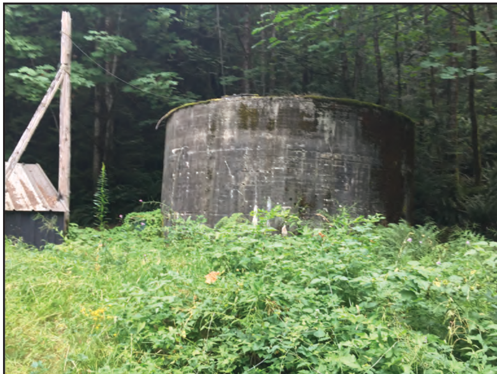
Figure 12: Phase IV Tank, facing north by northeast.
