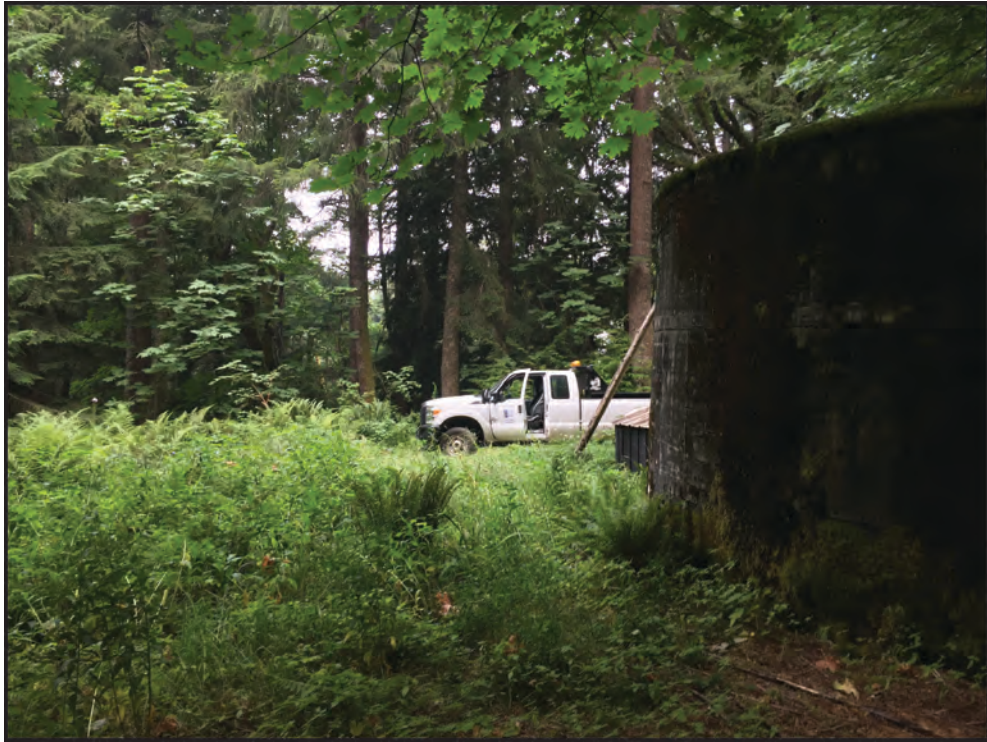
Figure 14: Phase IV Tank, facing west.
