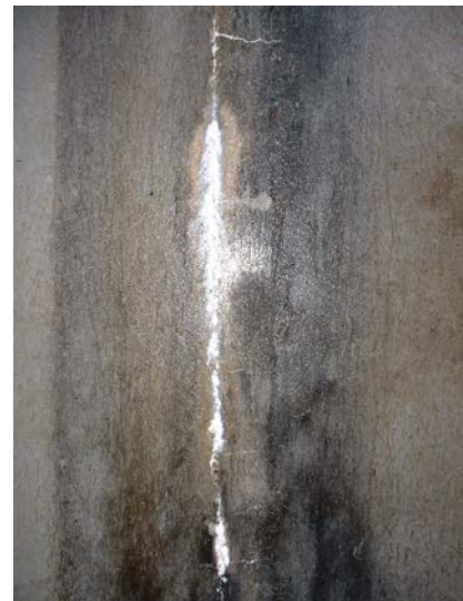
54. Horizontal and vertical cracks adjacent to north west anchor blocks
