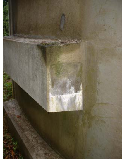
52. Note efflorescence at SE anchor block
