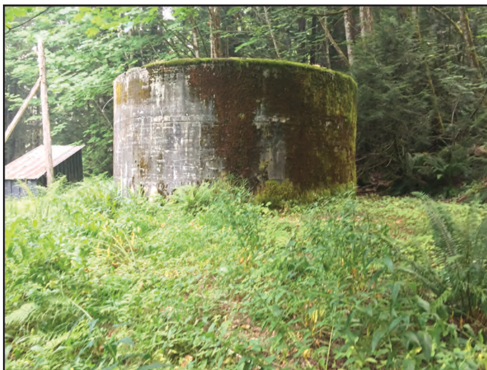
Figure 13: Phase IV Tank, facing north.
