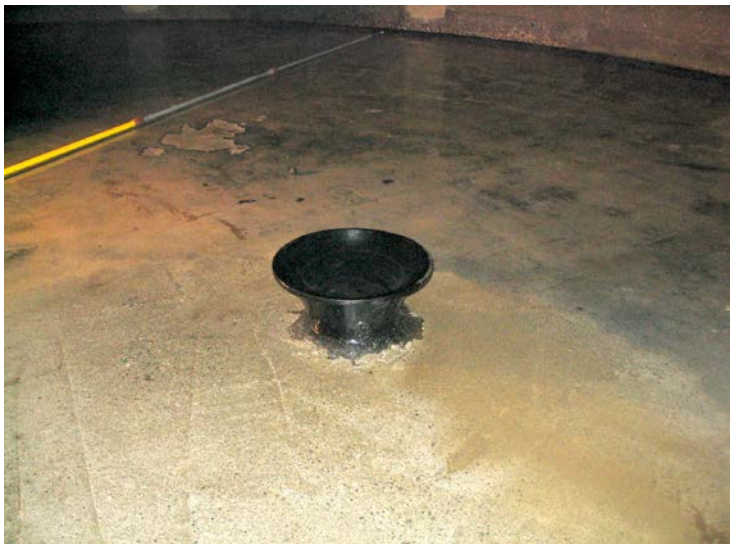
144. 250 Φ bellmouth inlet drain
