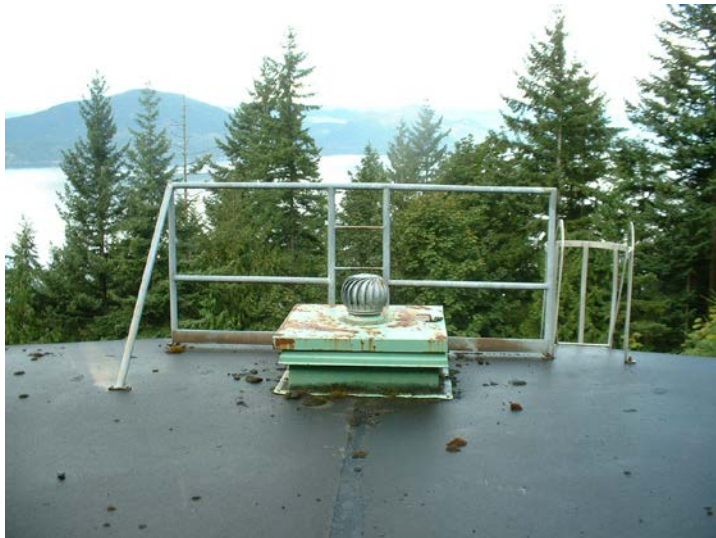
57. Roof hatch and vent
