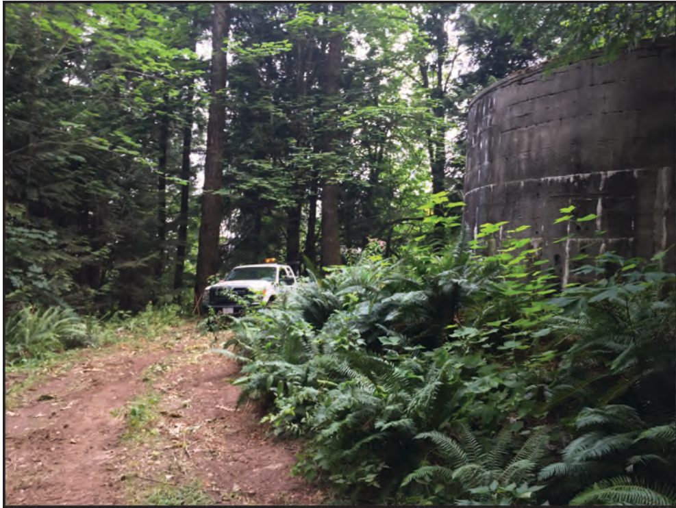
Figure 16: Phase V Tank, facing north by northwest.
