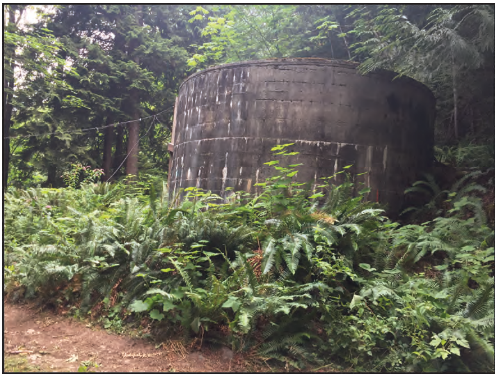
Figure 15: Phase V Tank, facing north.
