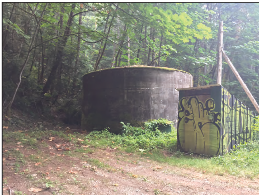
Figure 11: Phase IV Tank, facing southeast.
