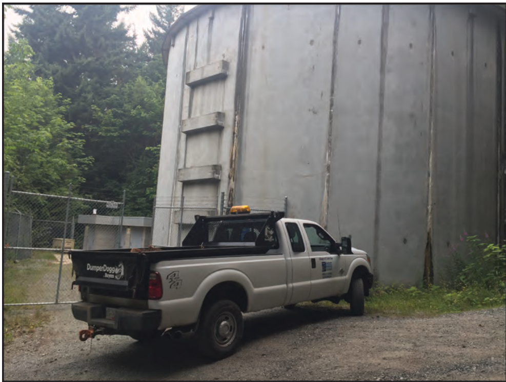
Figure 19: Harvey Tank, facing north by northwest.
