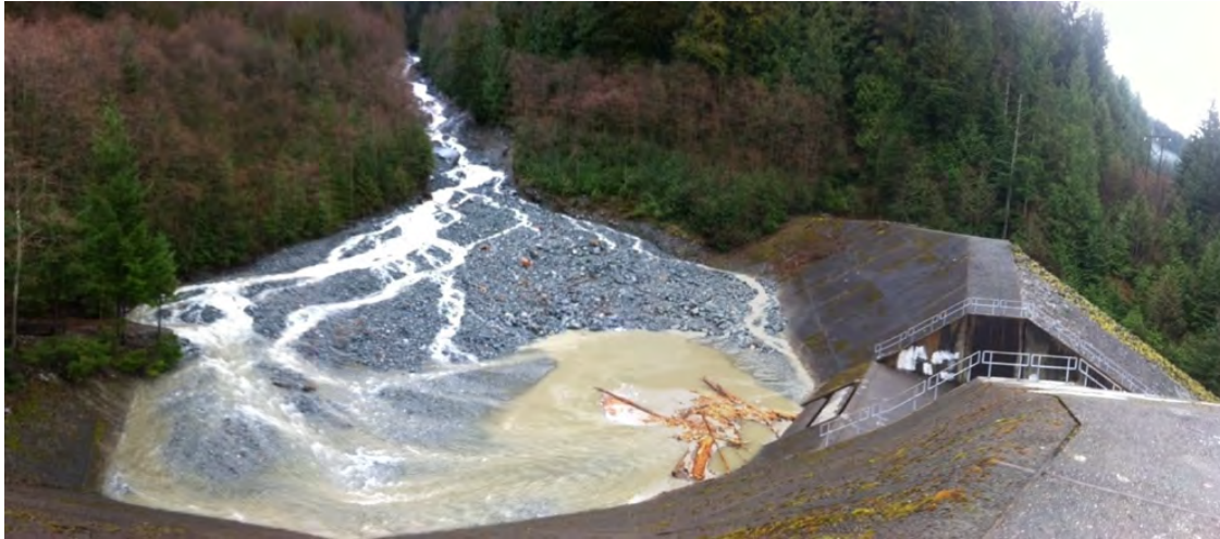
Figure 3. Charles Creek retention structure with debris flow infill. Downloaded from internet ( https://www.flickr.com/photos/tranbc/8510095573 ).
