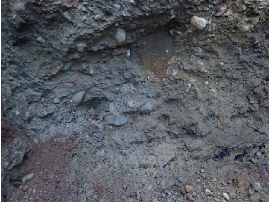
Photo 1. Till in house excavation, Lot 60 Oceanview Road.
