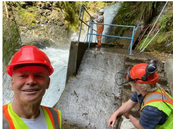
Picture: Mayor Berry and Team at water intake
