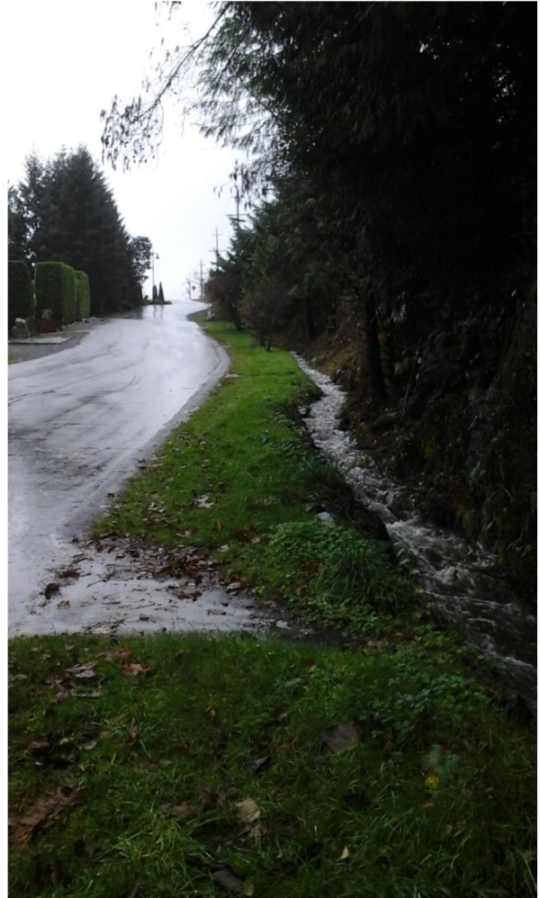
Figure 4-4: Photos of Roadway Ditch
