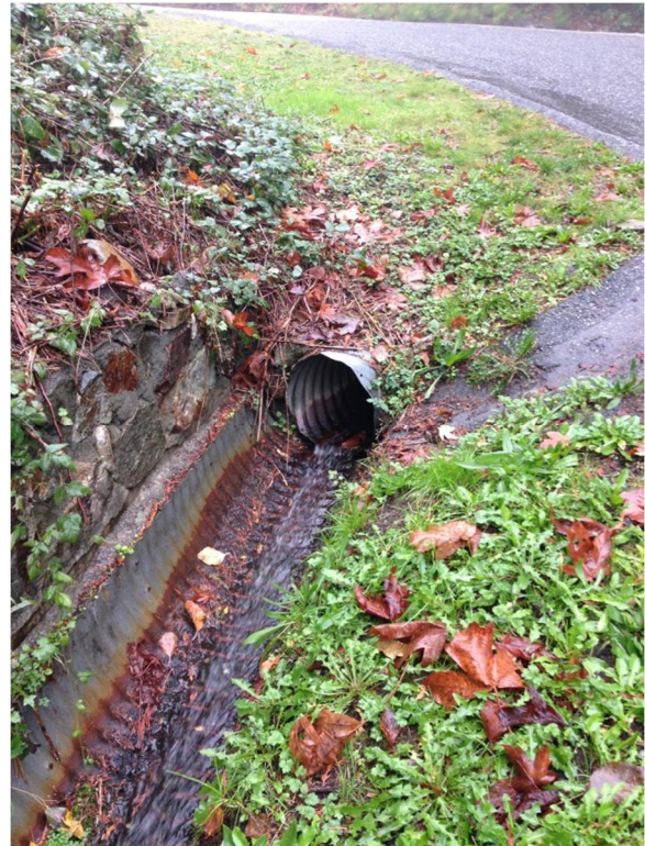
Figure 4-2: Photo of Corrugated Steel Pipe Culverts
