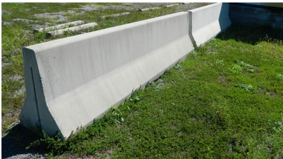
Example of Jersey Barrier
