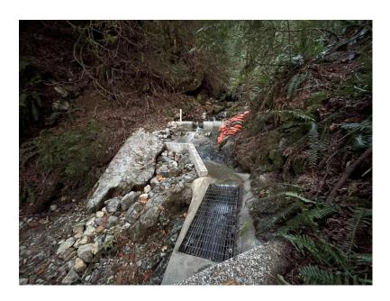
The municipality monitors creek flow continuously, using solar-powered cellular-connected depth sensors in the whole-stream pools above the Harvey and Magnesia creek intake weirs. Last week saw midday creek flow peaks flattening out, implying that daytime snowmelt is no longer a significant source of supply. Organics loadings increased at the same time, as expected when supply moves to groundwater only; chlorine dosing has been increased as necessary.
