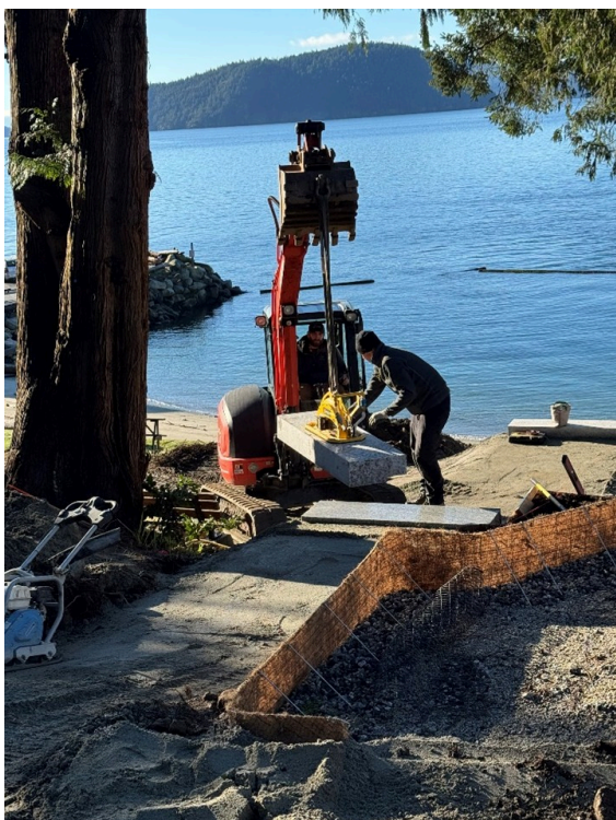
Installation of New Granite Stair Treads
